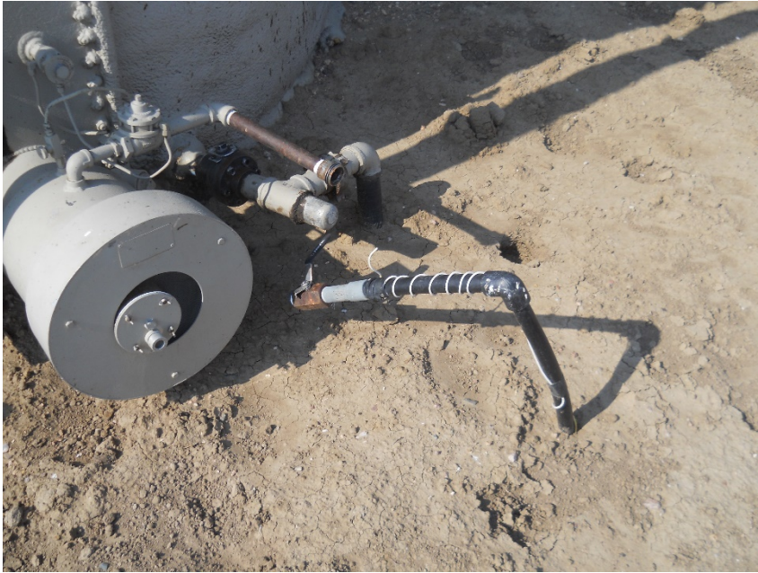
1" unused poly riser north side of east crude tank
