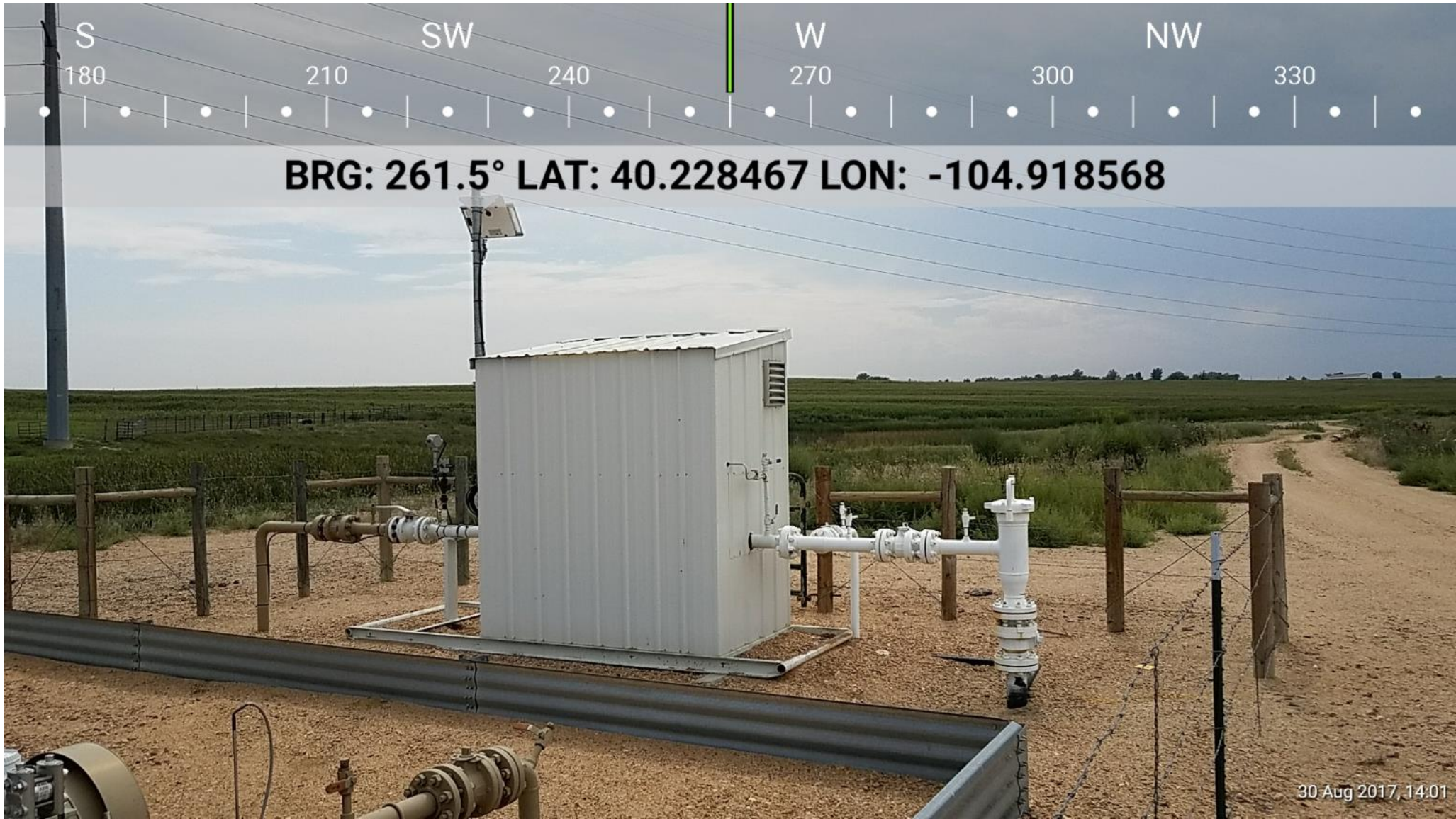
Gas Meter Run and Pig Station
