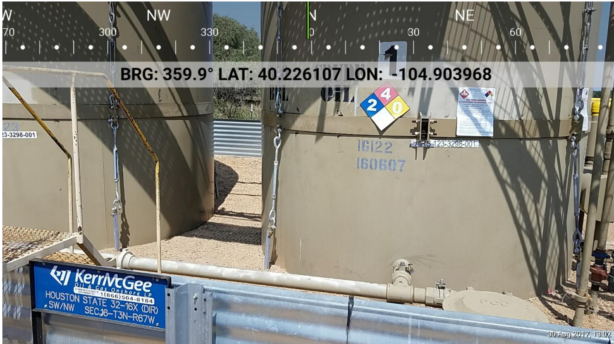
Flood Anchoring on Crude Tanks
