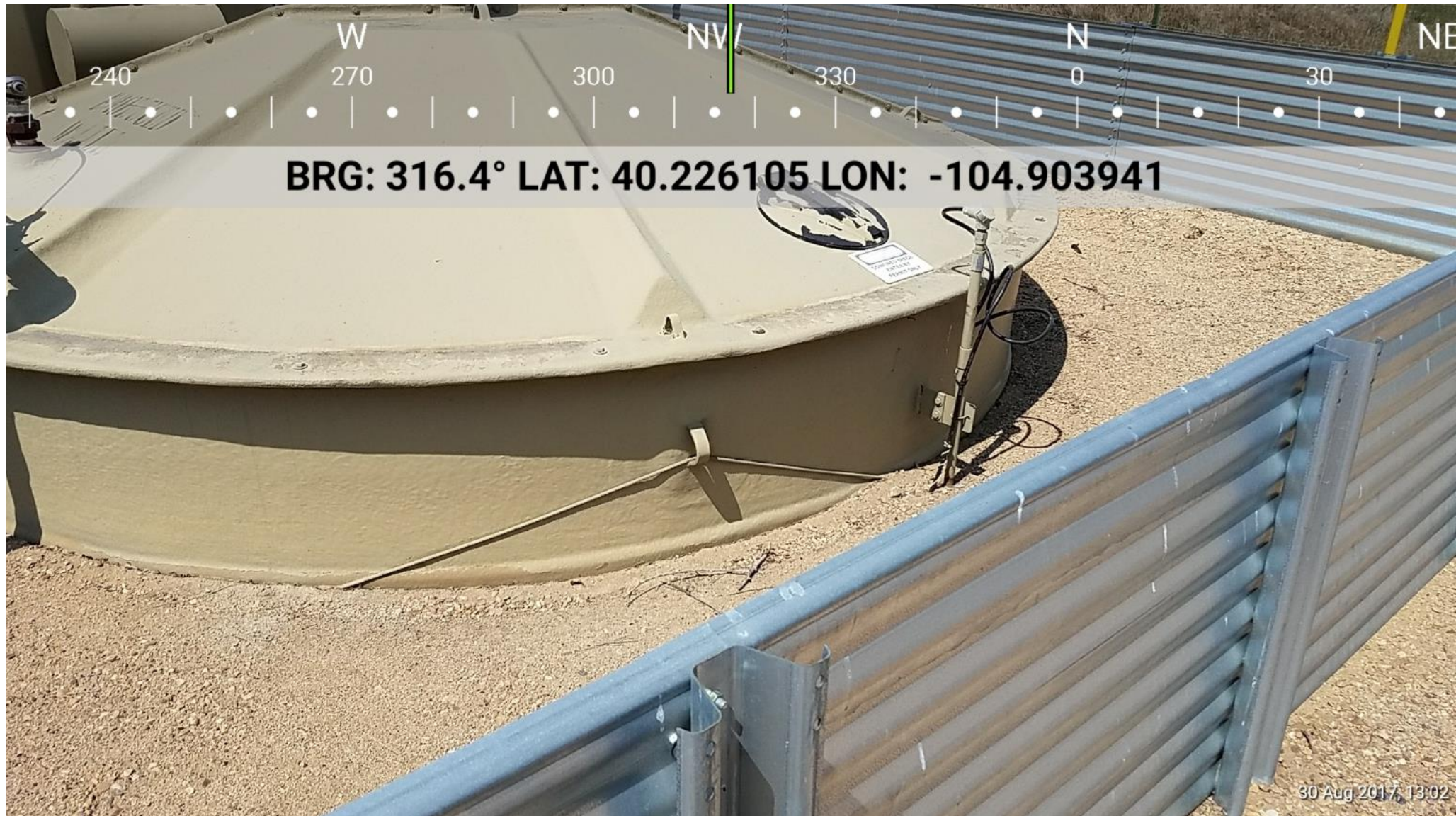
Flood Anchoring on Produced Water Tank Location #: 330428
