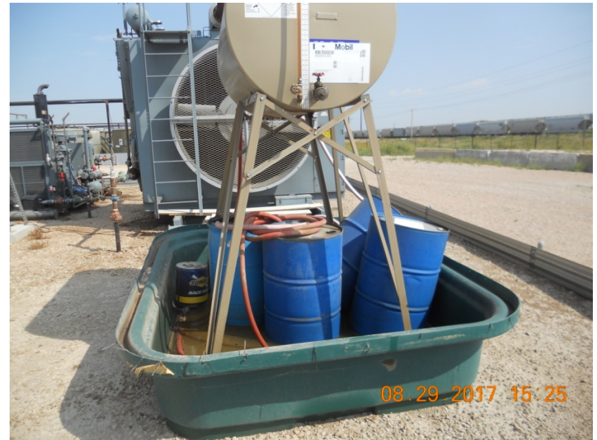
Photo 2. No Net oil containment , no liquids observed
