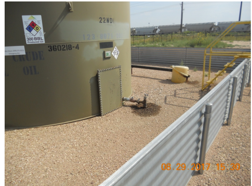
Photo 2. No Net oil containment , no liquids observed
