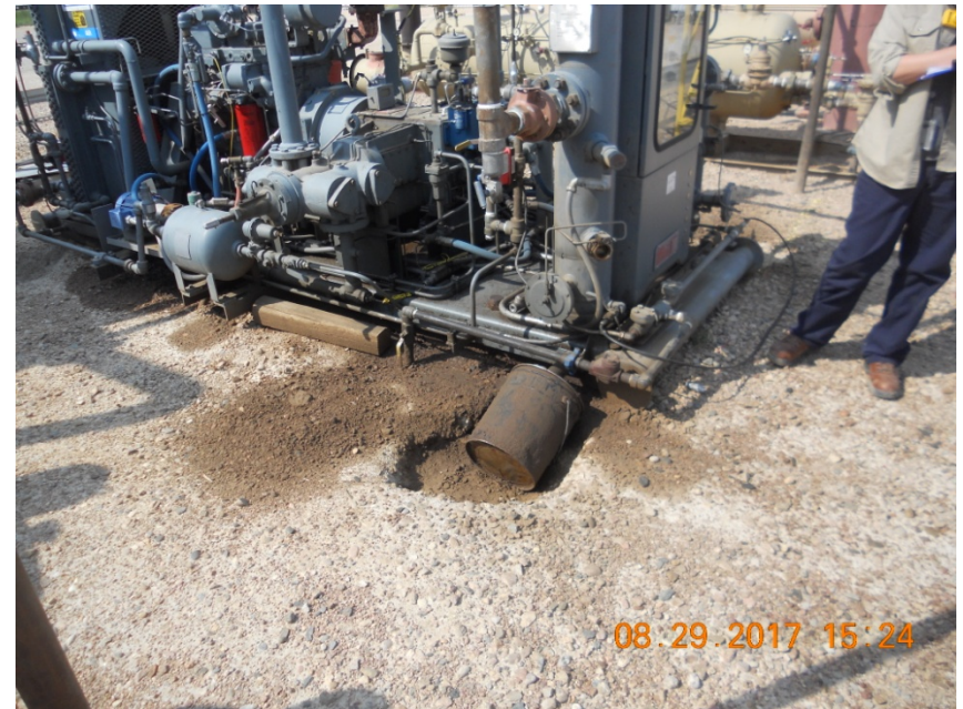
Photo 2. No Net oil containment , no liquids observed
