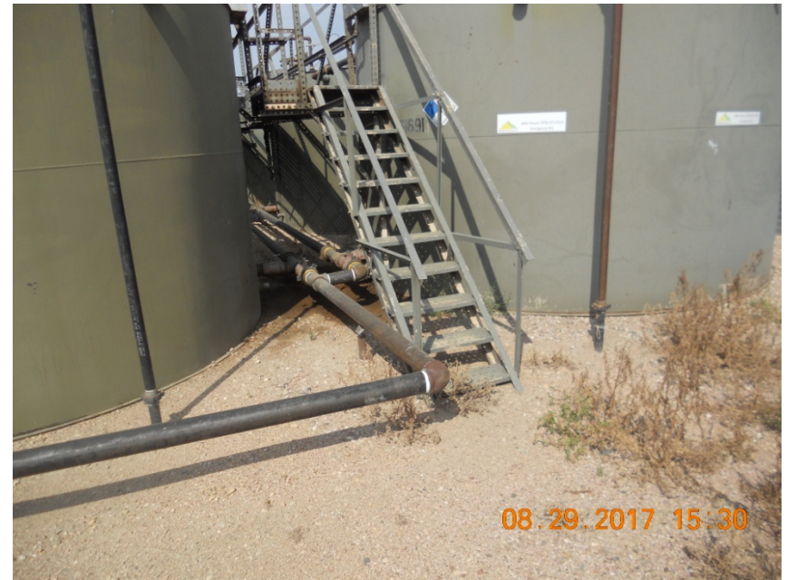
Photo 2. No Net oil containment , no liquids observed
