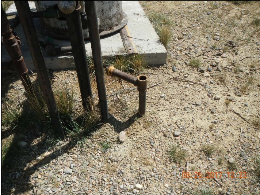
Photo 5. 2" steel riser not marked for abandonment or locked out tagged out.
