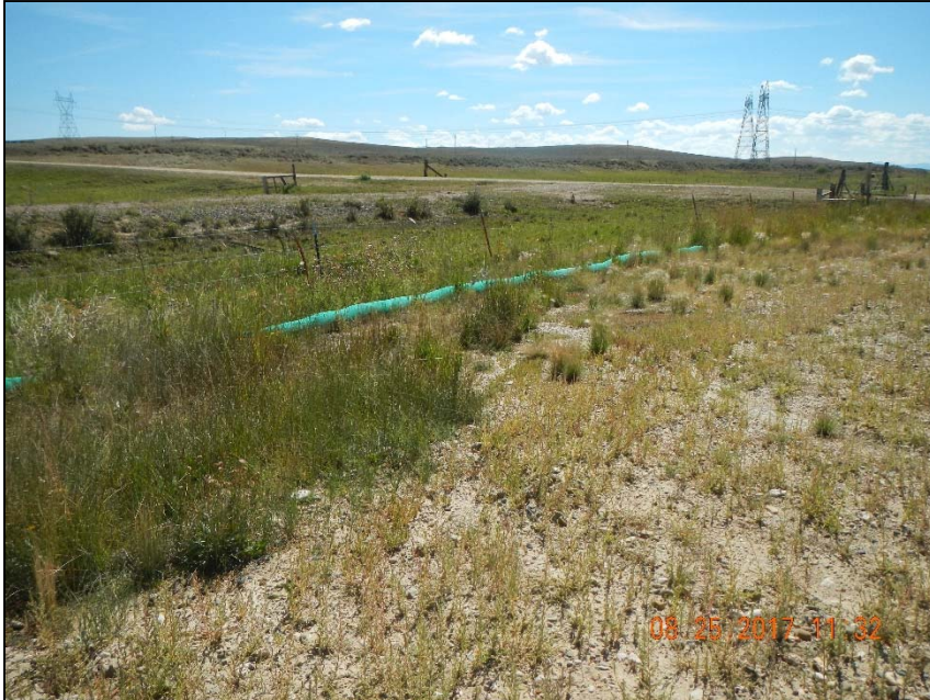
Photo 5. Inadequate stormwater BMP and maintenance.
