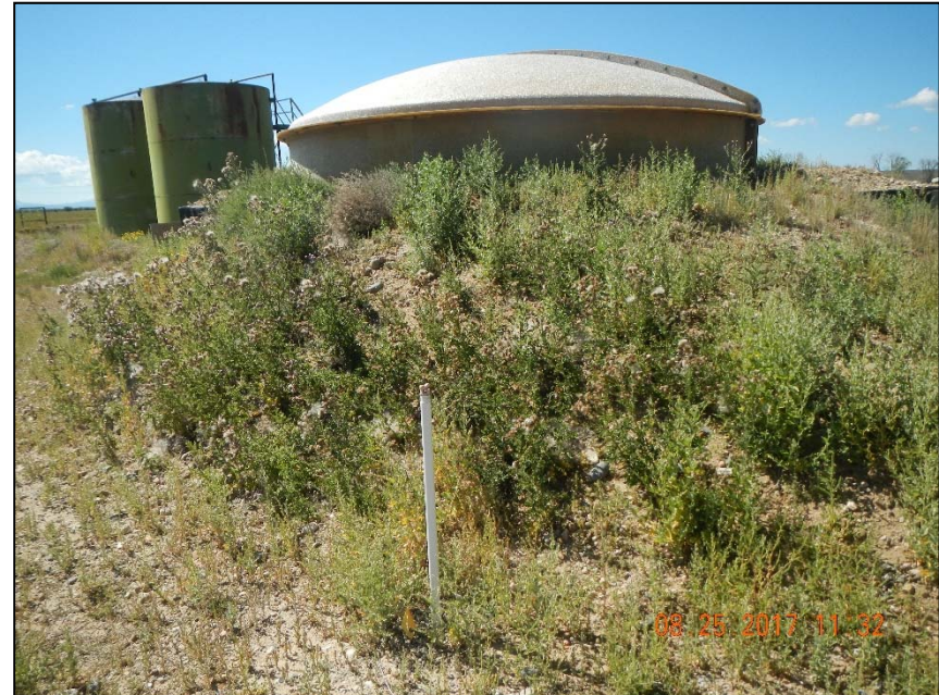
Photo 4. Fiberglass tank with no berm.
