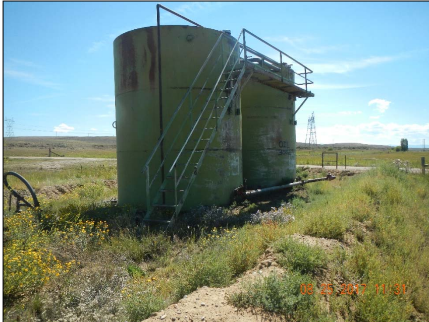
Photo 3. Weeds and vegetation in tank berm.
