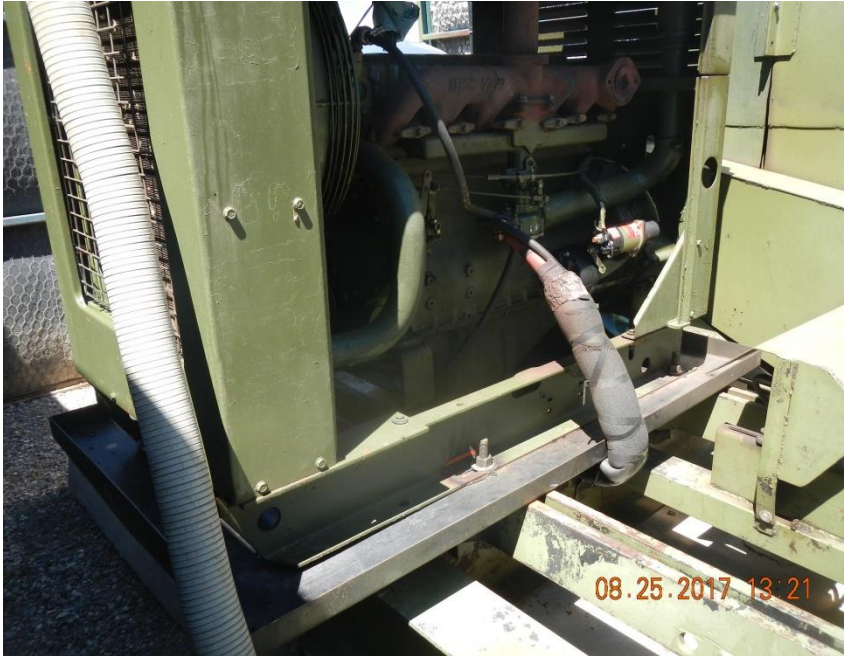
Drip pan for prime mover engine.
