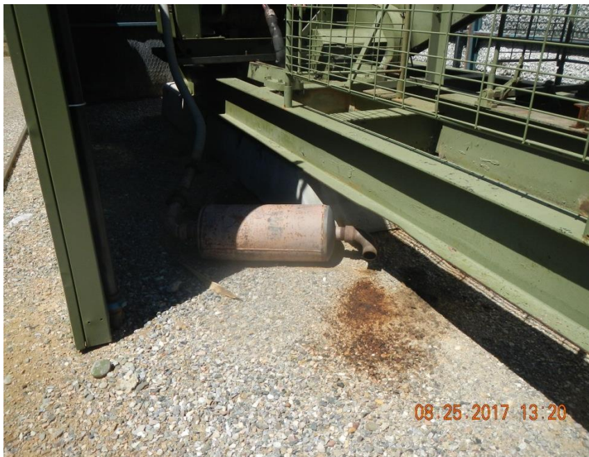
Stained soil beneath prime mover exhaust.
