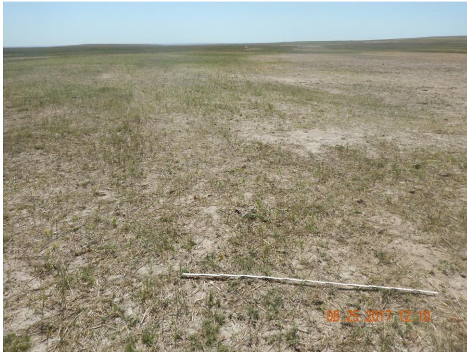
Photo 3: Photo taken from the former battery location, facing south. Photo shows erosion has been repaired, areas had been seeded with an oat grass species, and straw crimped to stabilize the site.
