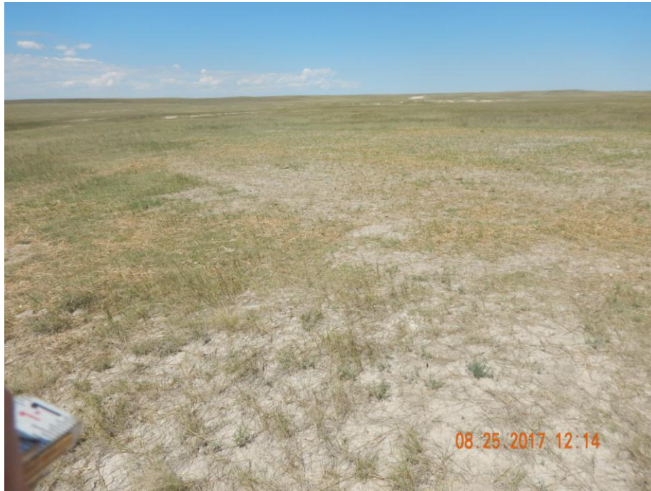
Photo 5: Photo taken the south end of the well location, facing north. Photo shows areas had been seeded with an oat grass species, and straw crimped to stabilize the site.
