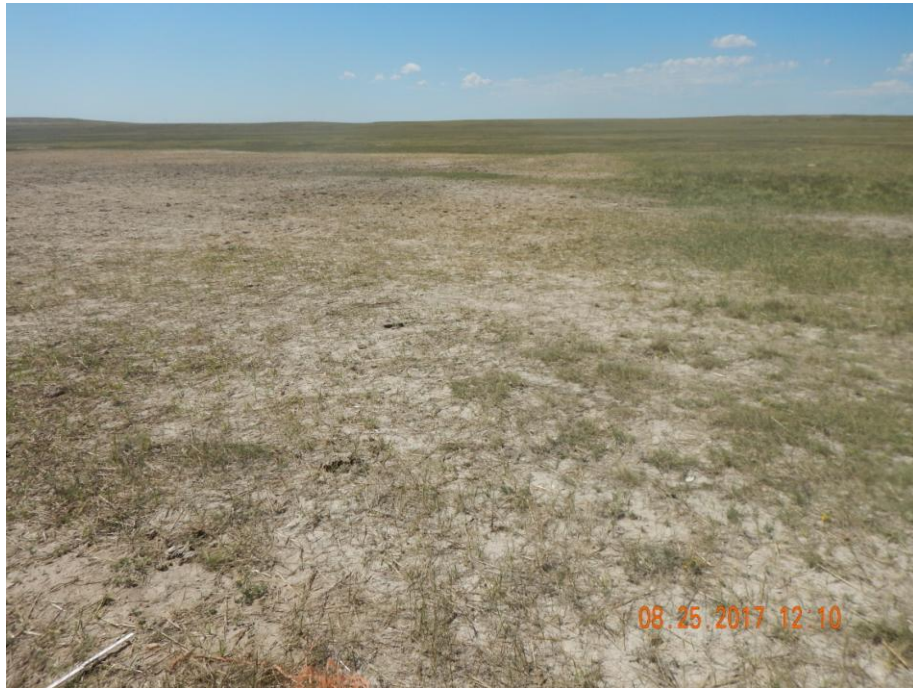
Photo 5: Photo taken from the former battery location, facing west. Photo shows erosion has been repaired, areas had been seeded with an oat grass species, and straw crimped to stabilize the site.
