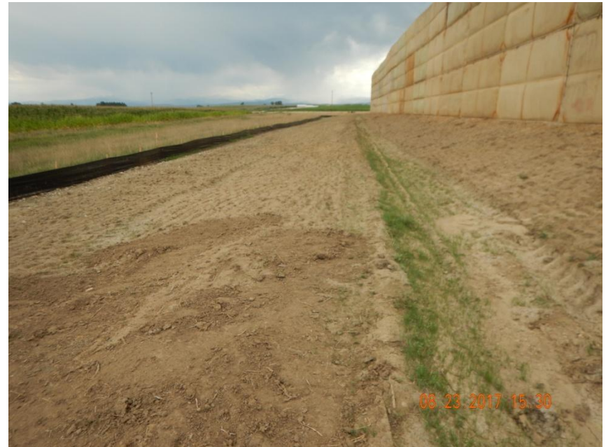
Photo 4. Photo taken from the south-central location, facing West. Silt fence BMP installed around the western and southern location. Silt fence BMP installed around the western and southern location. A ditch BMP was observed just below the base of the well pad and the southern slope has been tracked perpendicular with equipment.
