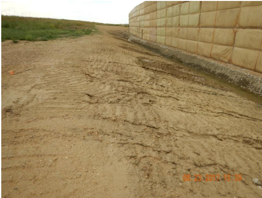
Photo 11. Photo taken from the northwestern location, facing East. Rill erosion starting to develop along the portions of the cut slope. Did not observe any BMPs to manage and control for stormwater run-on onto location. Additional BMPs to manage and control for stormwater run-on onto location should be installed so the northern cut slope can be stabilized.
