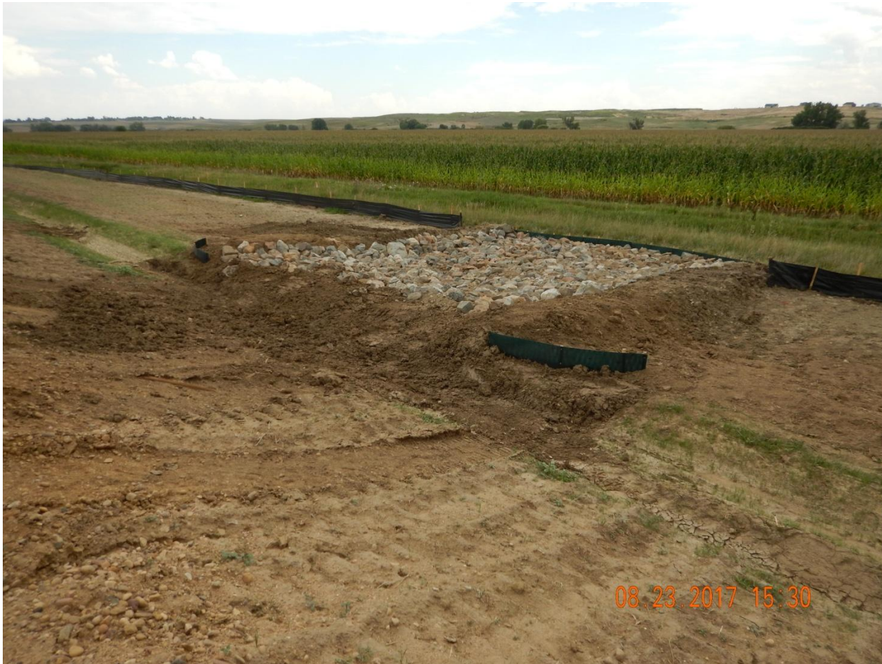
Photo 5. Photo taken from the south-central location, facing Southeast. A stabilized area constructed of rip-rap has been installed to for erosion control. The outlet of the rip-rap has been installed with S-Fence for sediment control- see next photo.
