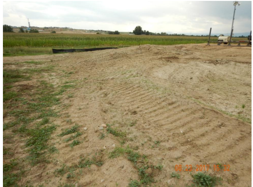
Photo 8. Photo taken from the southeastern location, facing South. Silt fence BMP ended at the southeast corner of the location. Did not observe any sediment or erosion control BMPs along the eastern perimeter of the location.
