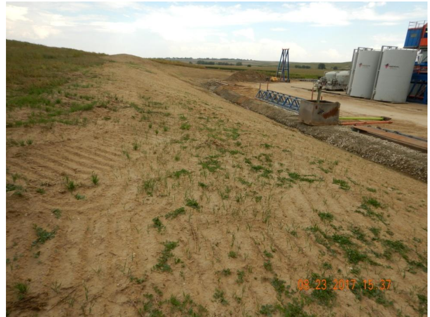
Photo 10. Photo taken from the northeastern location, facing East. The northern cut slope has been tracked perpendicular with equipment for temporary stabilization. Did not observe any BMPs to manage and control for stormwater run-on onto location. Rill erosion starting to occur along the northwestern cut slope- see the next photo.
