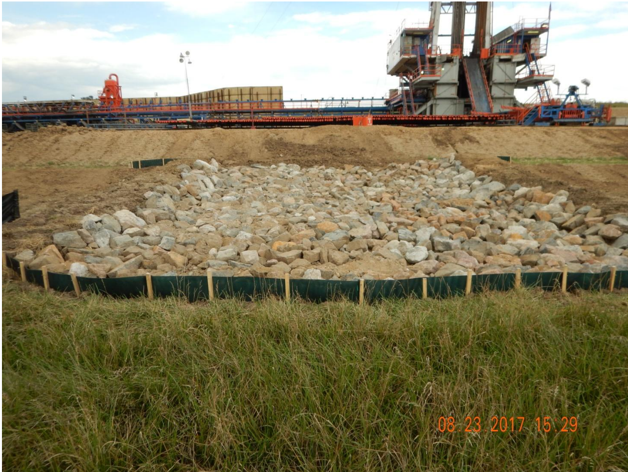
Photo 6. Photo taken from the outlet area of the stabilized rip-rap area, facing North. S-Fence has been installed for sediment control.
