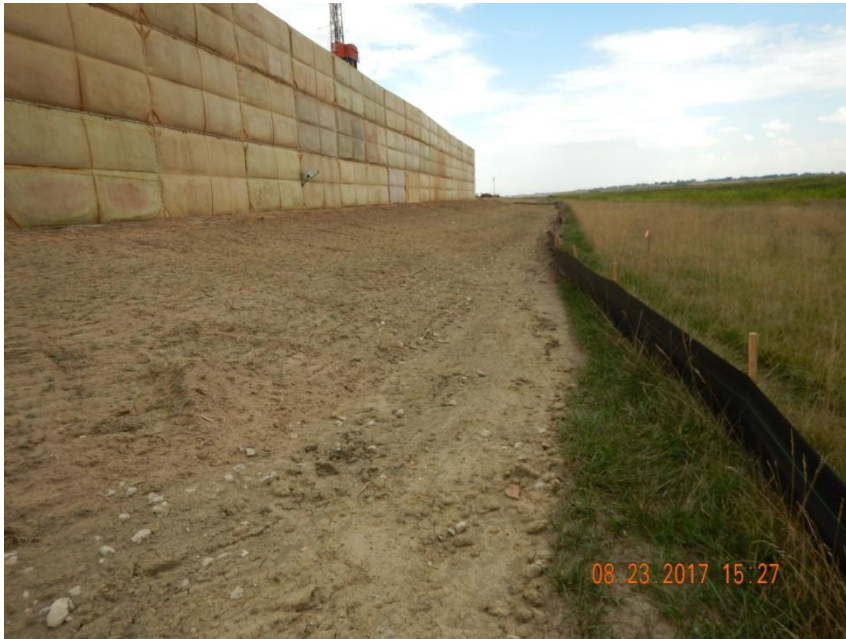
Photo 3. Photo taken from the southwest location, facing East. Tracking pad devices installed at location. Silt fence BMP installed around the western and southern location. A ditch BMP was observed just below the base of the well pad and the southern slope has been tracked perpendicular with equipment.
