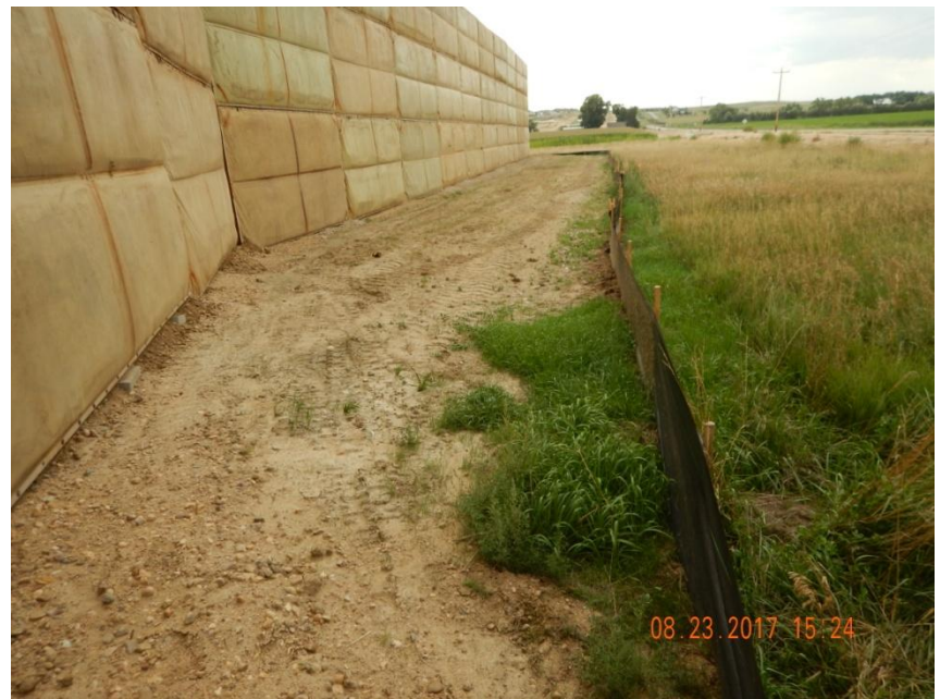
Photo 2. Photo taken from the western location, facing South. Silt fence BMP installed around the western and southern location.
