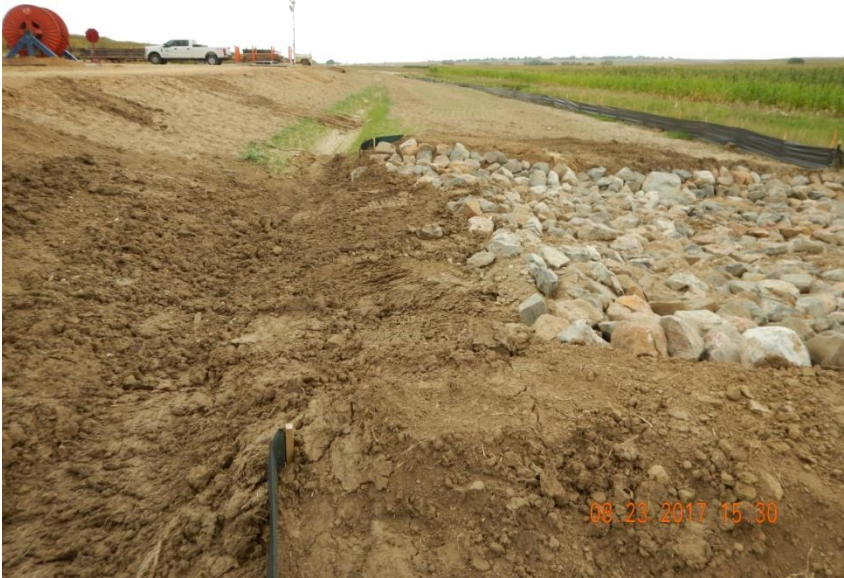
Photo 7. Photo taken from the stabilized area, facing East. Silt fence BMP installed around the western and southern location. A ditch BMP was observed just below the base of the well pad and the southern slope has been tracked perpendicular with equipment.
