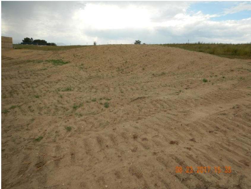
Photo 9. Photo taken from the northeastern location, facing Northwest. Appears to be the topsoil stockpile which has been temporarily stabilized.
