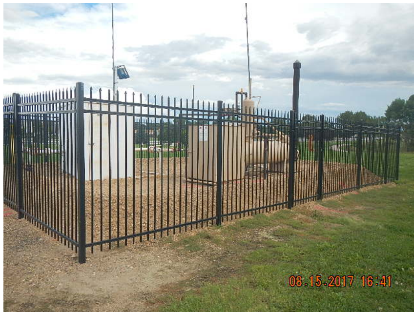
Separator taken from NW
