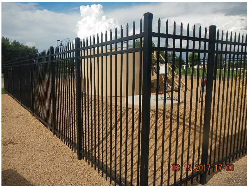
Tanks and berms taken from SW
