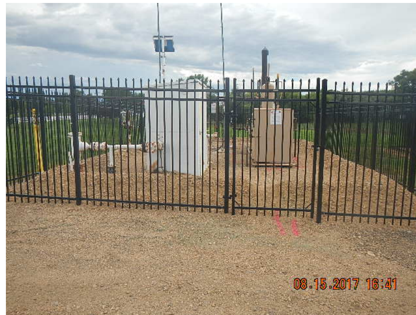
Separator taken from the North
