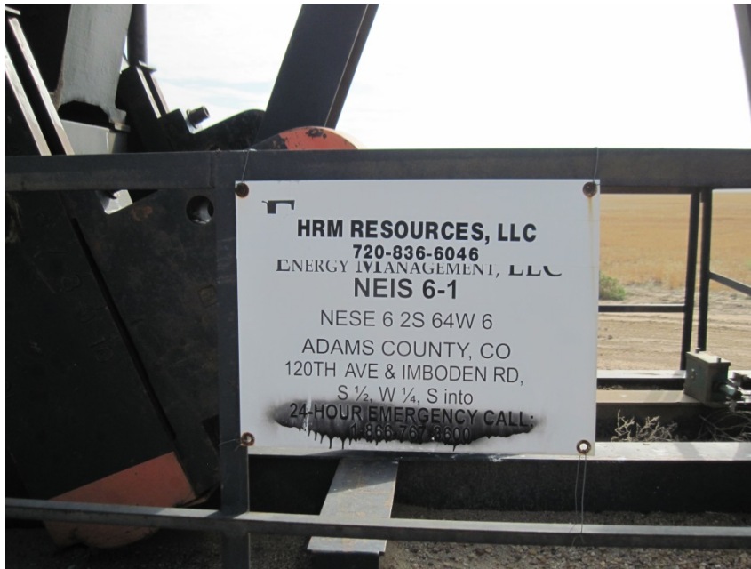
WELLHEAD AND PUMP JACK
