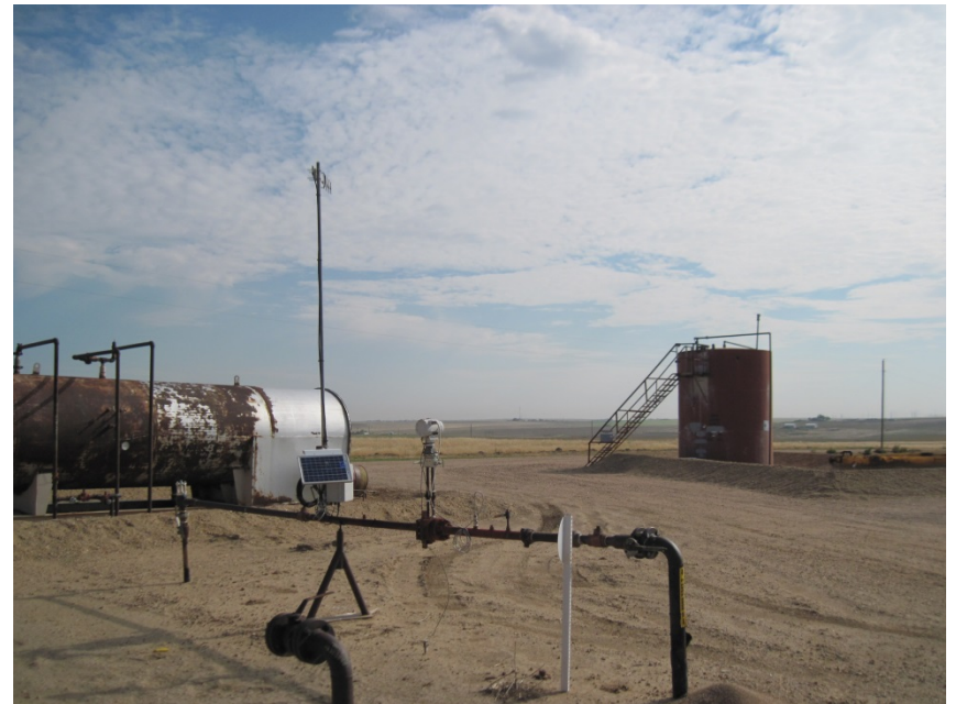
PRODUCTION EQUIPMENT AND BATTERY
