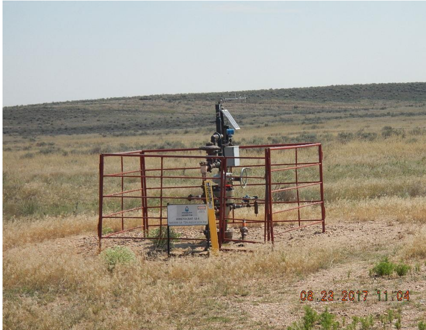
Photo 1 Wellhead from west
