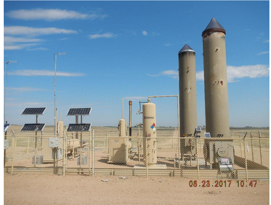
Photo 2: Separators/ECB from south
