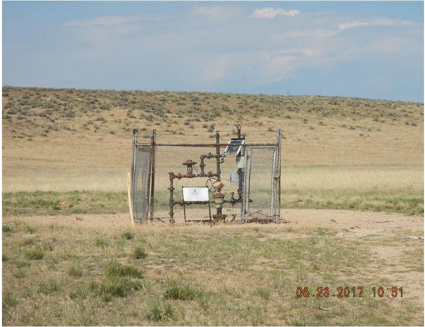
Photo 4: Wellhead from east
