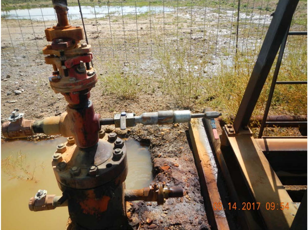
1" port after install of blind plug and additional valve.
