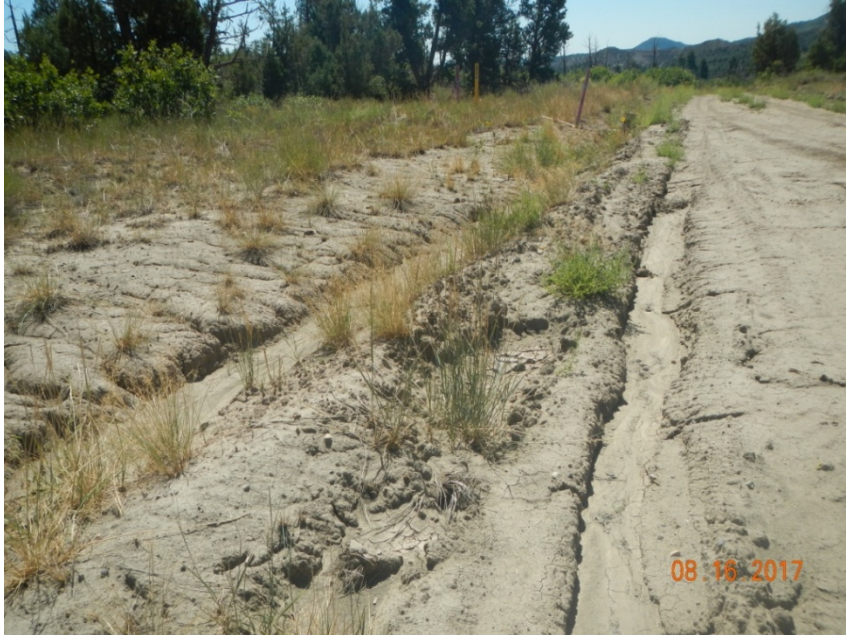
Photo 7: View of erosional downcutting and unstabilized soils near the well pad entrance facing eastward.
