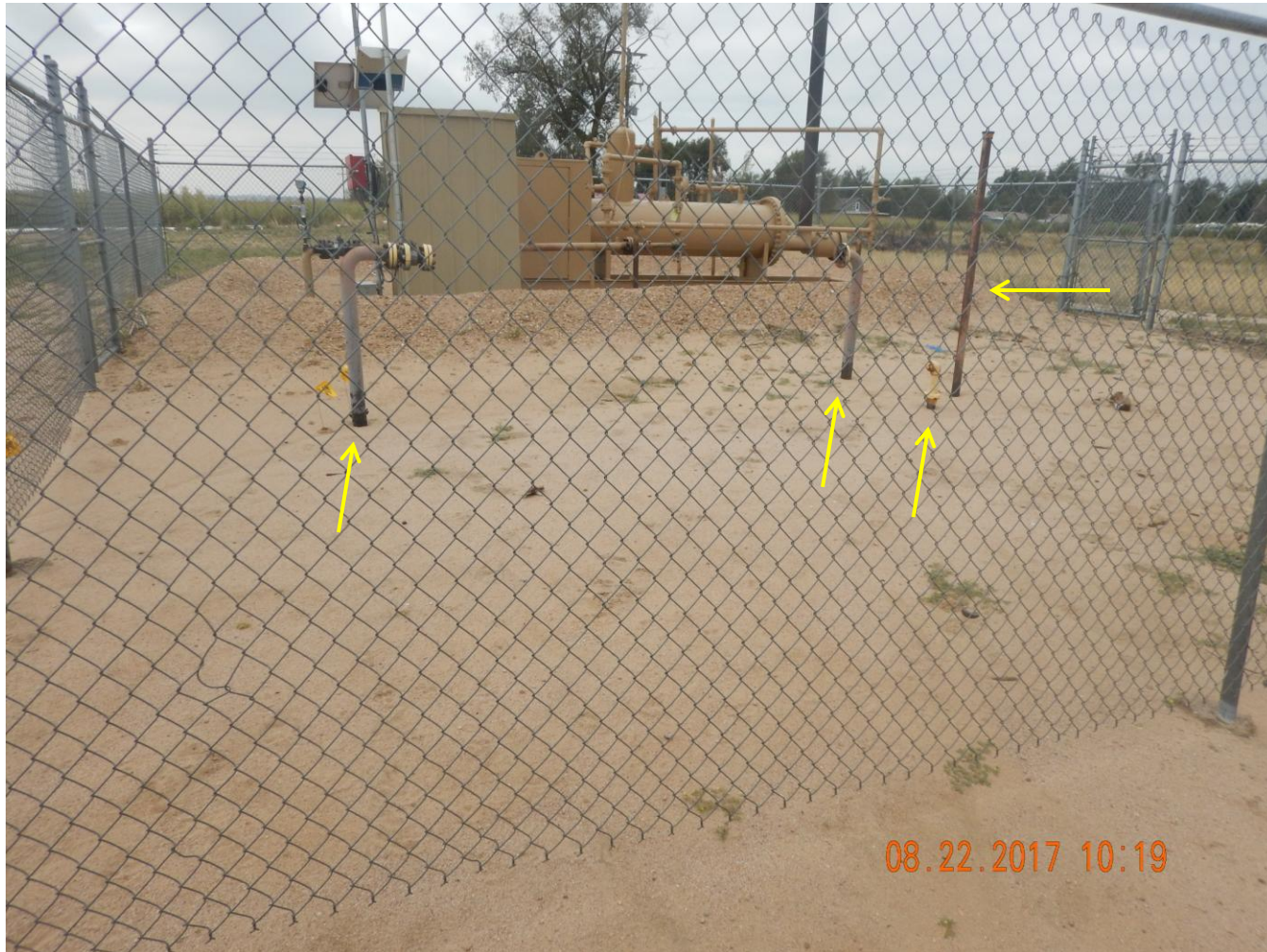
Photo 5: Photo taken from the east end of the battery facility location, facing south. Inspection doc. #682502476 identified four (4) risers at the battery location, and required they be removed in accordance to 1004.a. Photo shows risers have not been removed.
