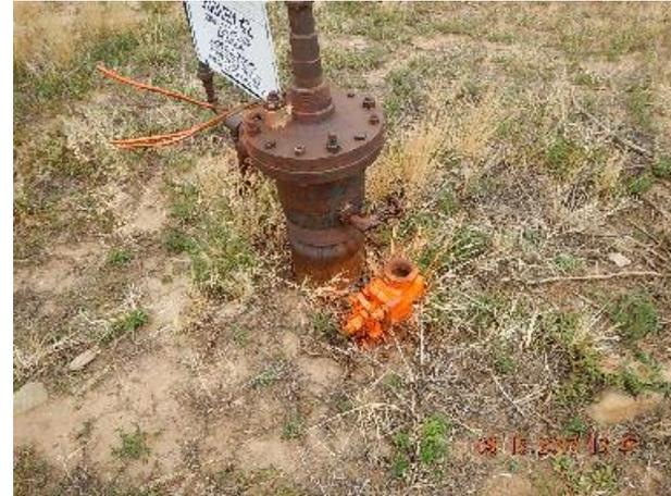
Photo 2: Riser at wellhead.
