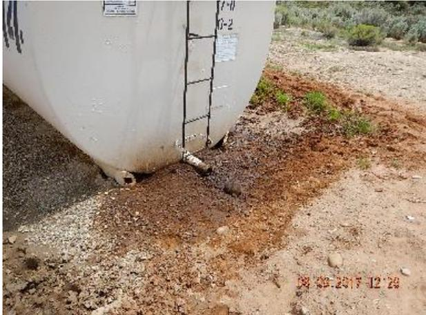
**Photo 5: Production tank with broken nipple and released oil inside containment.**
