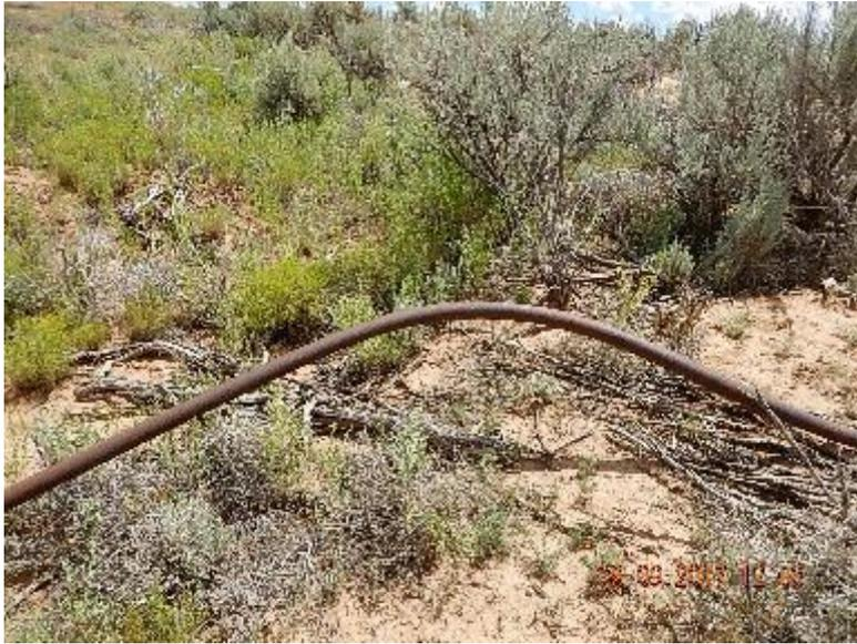
**Photo 1: Steel line – disconnected and open on both ends.**
