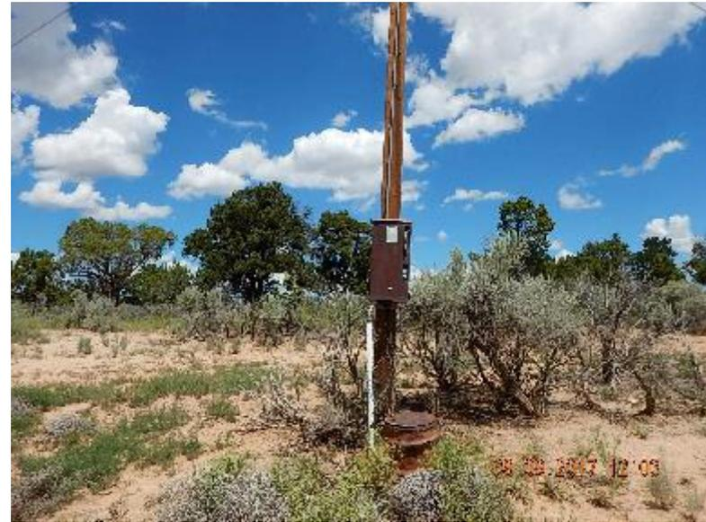
Photo 4: Electrical service panel and power pole.
