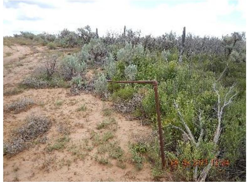
**Photo 2: Disconnected 1" steel line.**
