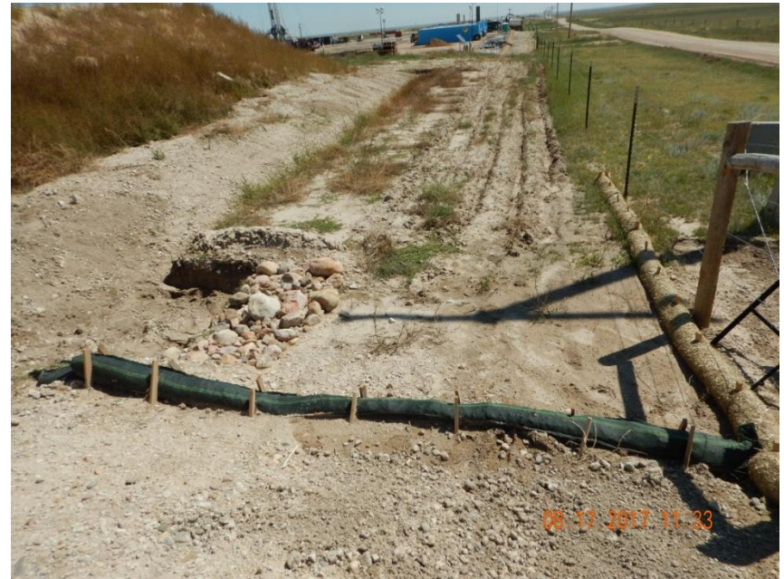
Photo 8. Photo taken from the entrance of the east Holliday entrance, facing East. Sediment trap does not appear to be a sufficient size and does not appear to be constructed with good engineering practices.
