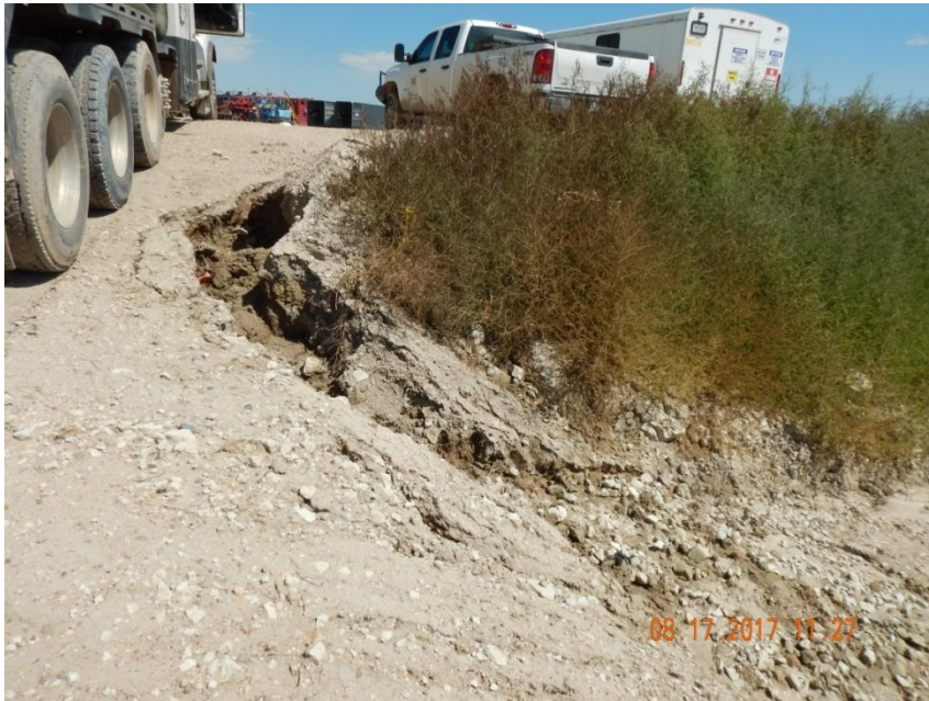
Photo 3. Photo taken from the previously mentioned gully erosion along the entrance of the Tombstone pad, facing Northeast.
