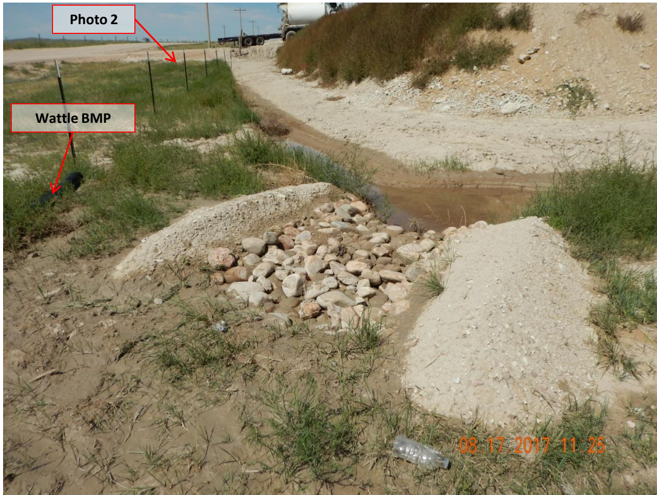
Photo 1. Photo taken from the southeast Tombstone pad, facing West. Sediment discharge observed beyond the outlet area of the sediment trap as shown in this photo. Does not appear the wattle BMP beyond the outlet area of the sediment trap is preventing sediment discharge from location. Sediment trap has not been enlarged since the previous inspection on July 11, 2017.
