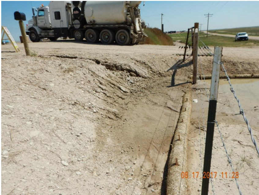
Photo 5. Photo taken from the entrance of the Tombstone pad, along the west side, facing East. Gully erosion occurring along the west entrance access road. Wattle BMPs are not preventing sediment discharge from location.
