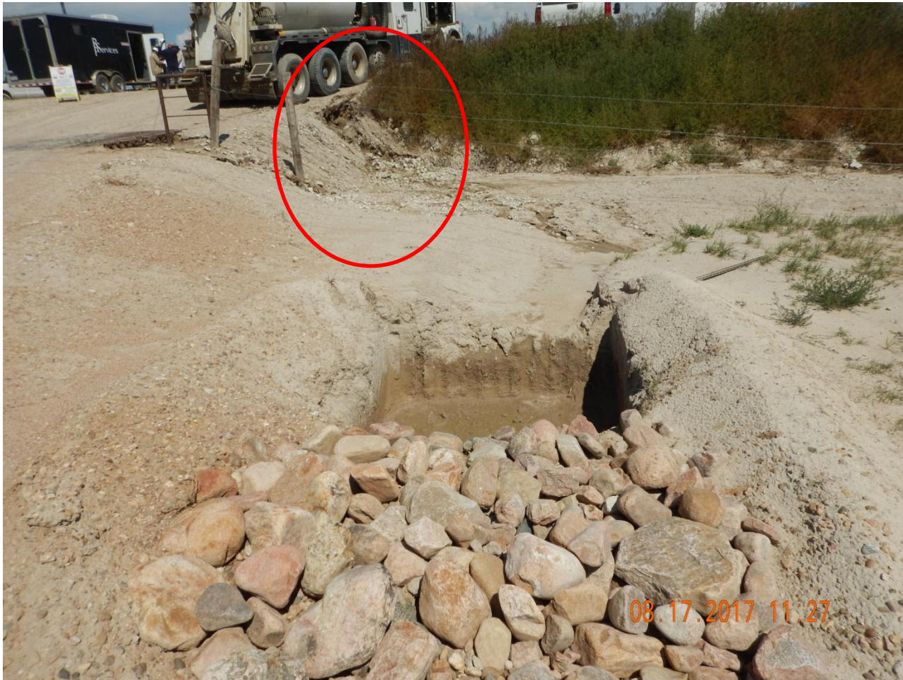
Photo 2. Photo taken from the entrance of the Tombstone pad, along the east side, facing North. Sediment trap has been installed to capture stormwater runoff from the access road. Gully erosion occurring along the east access road entrance (red circle)- refer to Photo 3.
