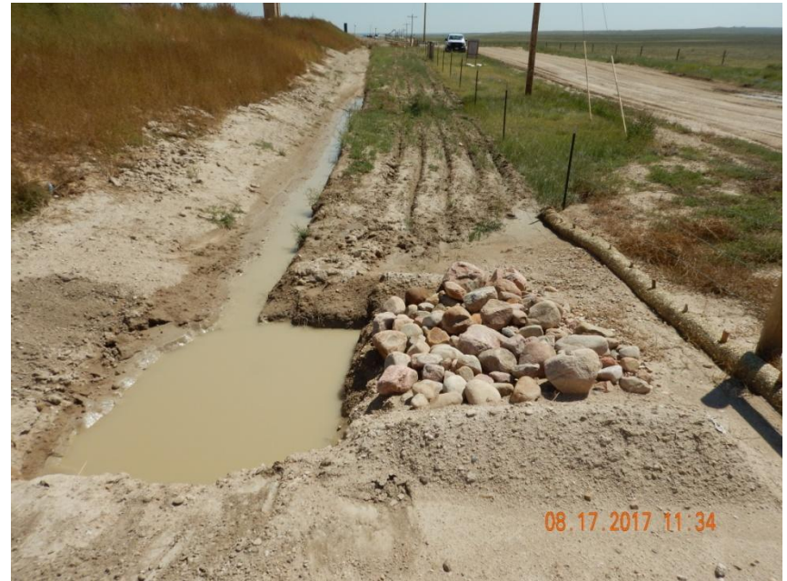
Photo 12. Photo taken from the entrance of the west Holliday entrance, facing East. Sediment trap does not appear to be a sufficient size. Appears flows have discharged over the embankment berms and around the outlet area.
