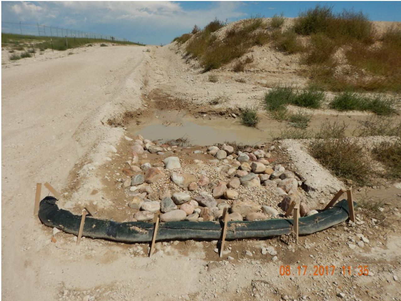
Photo 13. Photo taken from the southwest location of the Holliday pad, facing North. Sediment trap does not appear to be a sufficient size and does not appear to be constructed with good engineering practices. Sediment discharge was observed beyond the outlet area of the sediment trap.
