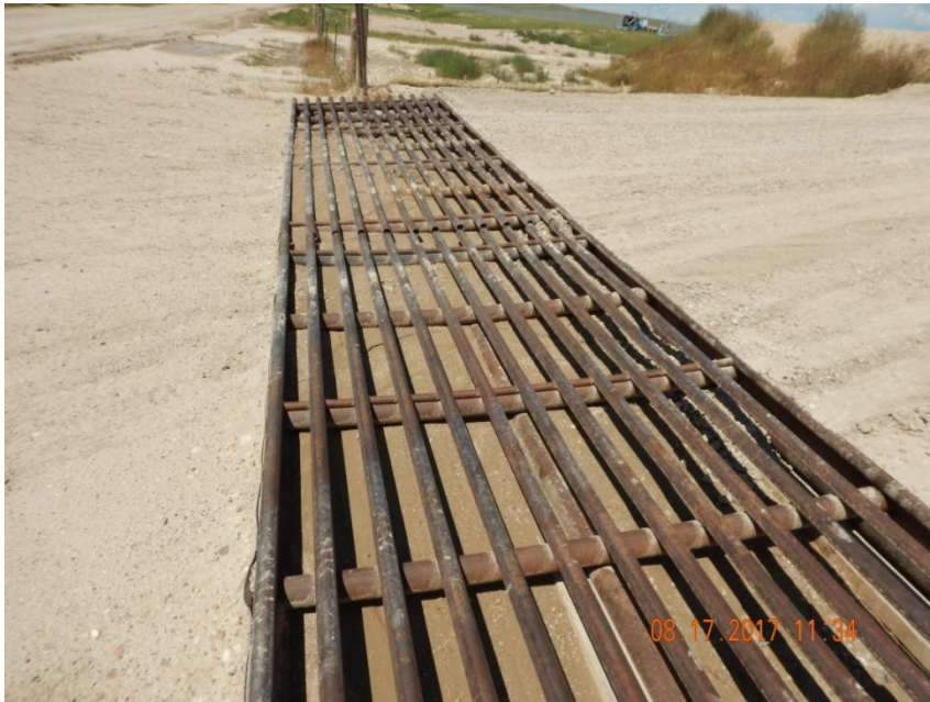
Photo 11. Photo taken from the cattle guard of the Holliday west entrance, facing West. Cattle guard in need of maintenance.
