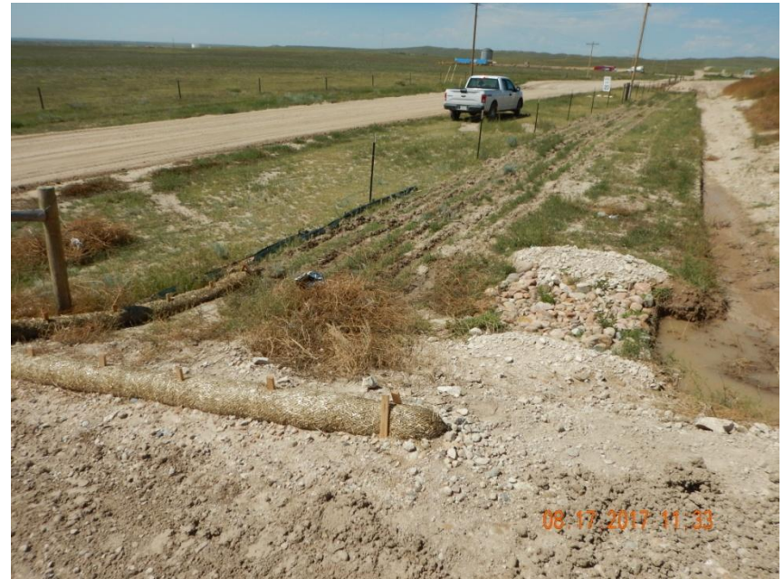
Photo 10. Photo taken from the previous photo, facing Southwest. Other BMPs (surface roughening and wattles) have been installed downgradient of the outlet area but may not be sufficient because the sediment trap appears too small.
