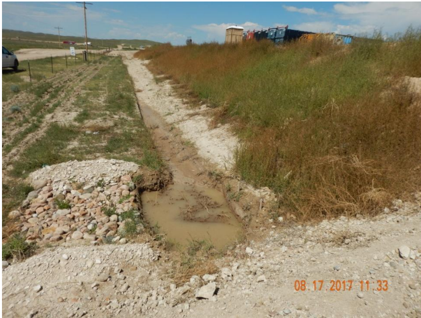
Photo 9. Photo taken from the entrance of the east Holliday entrance, facing West. Sediment trap does not appear to be a sufficient size.
