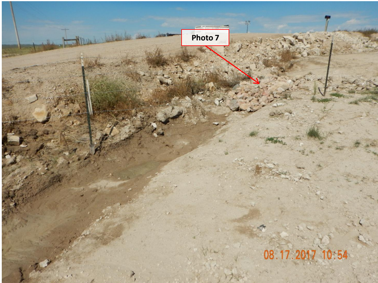
Photo 6. Photo taken from the ditch area between the two sediment traps, facing West. Operator has installed a shallow ditch from the outlet area of the upgradient sediment trap to the inlet area of the downgradient sediment trap. Ditch size may not be a sufficient depth to contain both outlet flows from the upgradient sediment trap and stormwater runoff from the access road.
