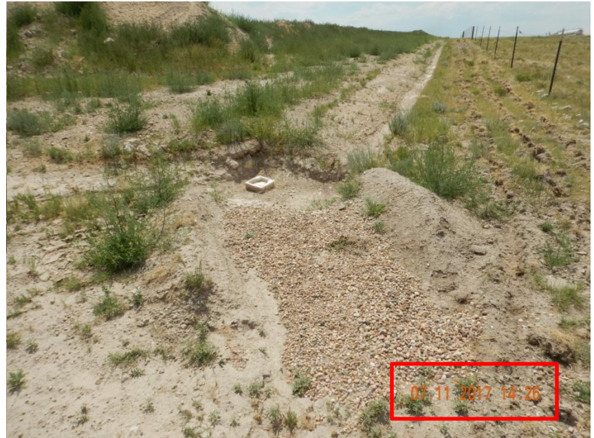
Photo 10. Photo taken of the sediment trap in Photo 9 from the July 11, 2017 inspection.
