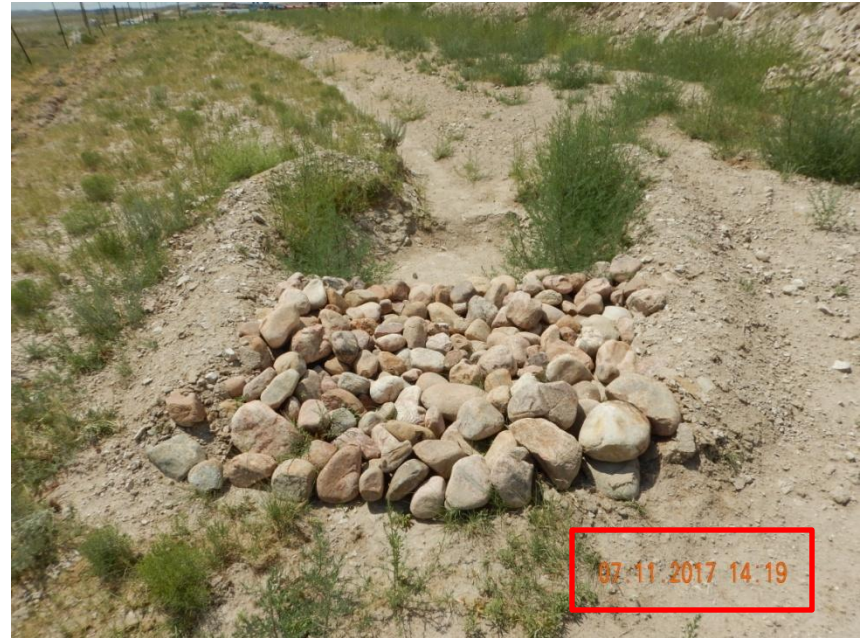
Photo 4. Photo taken of the sediment trap in Photo 3 from the July 11, 2017 inspection.
