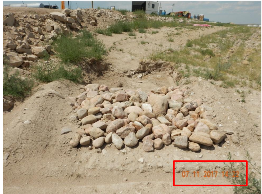
Photo 8. Photo taken of the sediment trap in Photo 7 from the July 11, 2017 inspection.
