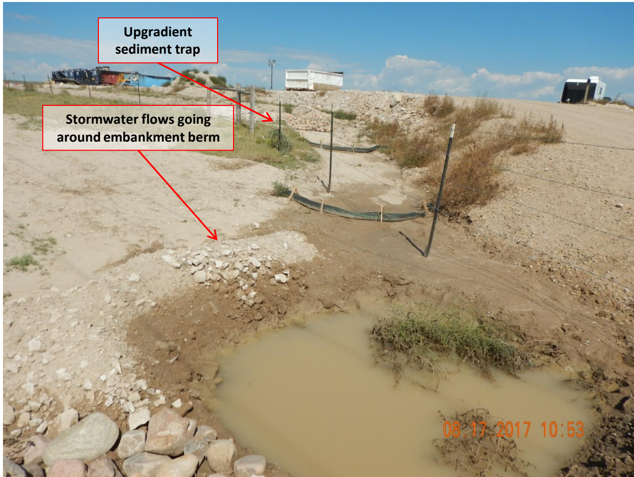
Photo 2. Photo taken from the previous sediment trap, facing North. Operator has installed a shallow ditch from the outlet area of the upgradient sediment trap to the inlet area of the downgradient sediment trap. Operator has installed filtrex wattles along the shallow ditch. Appears stormwater flows are going around the embankment berm of the downgradient sediment trap.
