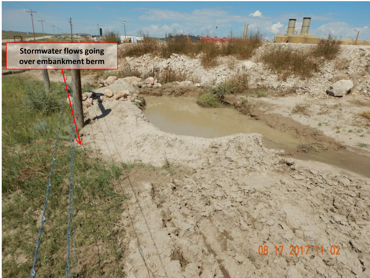
Photo 11. Photo taken from the southwest east well pad, facing West. Appears the Operator has enlarged the sediment trap size with two stabilized outlet areas. However, the sediment trap size could be enlarged because it appears flows have discharged over the embankment berms. Embankment material and embankment construction does not appear to be sufficiently compacted, as it appears unconsolidated material is contributing to sediment loss.
