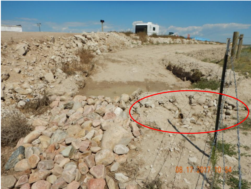
Photo 7. Photo taken from the previously mentioned upgradient sediment trap, facing Northwest. Appears the Operator has enlarged the sediment trap size with a stabilized outlet area. Embankment material and embankment construction does not appear to be sufficient compacted, as it appears unconsolidated material is contributing to sediment loss (red circle). Refer to Photo 8 for a picture taken of the sediment trap from the July 11, 2017 inspection.
