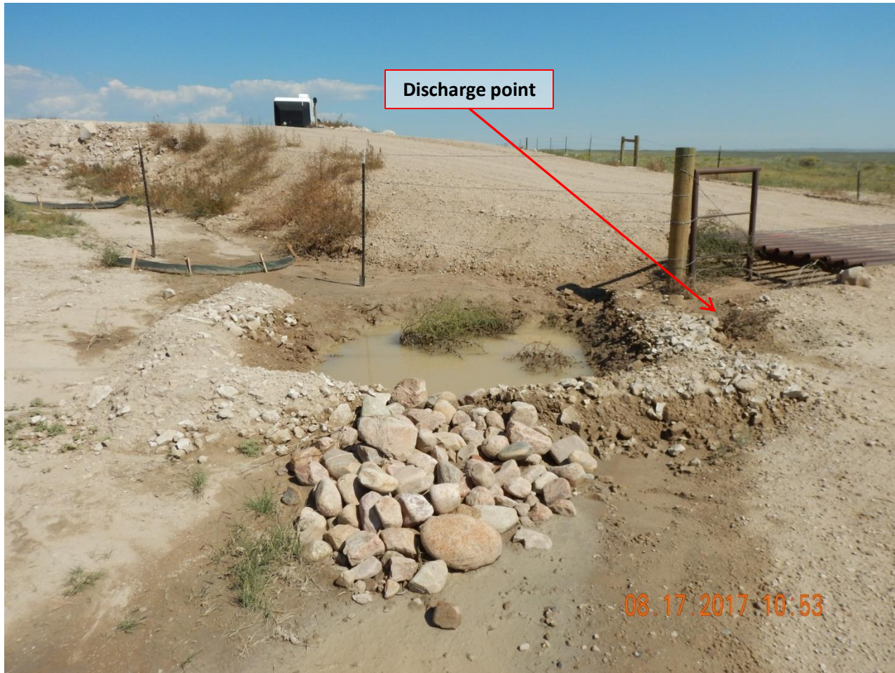
Photo 1. Photo taken from the east well pad, east entrance along the west side, facing Northeast. Operator has installed a second sediment trap near the entrance of the location. A discharge point was observed at the cattle guard as shown above. Embankment material and embankment construction does not appear to be sufficiently compacted, as it appears unconsolidated material could be contributing to sediment loss. Sediment trap outlet area does not appear to be properly constructed to capture outlet flows. Sediment trap size could be enlarged to help capture sediment laden stormwater runoff.
