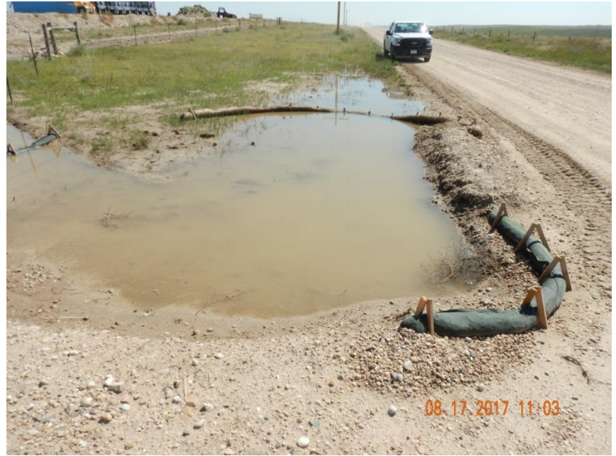
Photo 13. Photo taken from the previously mentioned shallow depression area, facing East. Does not appear the depression area with the wattles are pooling stormwater runoff. Appears the volume of stormwater sheet flow, likely sediment laden flow, is overtopping the wattle as shown in this photo.
