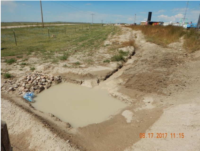
Photo 18. Photo taken from the west well pad, east entrance along the west side, facing West. Appears the Operator has installed a sediment trap. However, the sediment trap size could be enlarged because it appears flows have discharged over the embankment berms- see Photo 20. Embankment material and embankment construction does not appear to be sufficiently compacted, as it appears unconsolidated material is contributing to sediment loss. Refer to Photo 18 for a picture taken of this area from the July 11, 2017 inspection.
