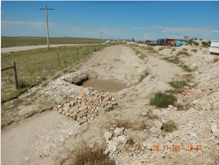
Photo 3. Photo taken from the previously mentioned upgradient sediment trap, facing West. Appears the Operator has enlarged the sediment trap size with a stabilized outlet area. Embankment material and embankment construction does not appear to be sufficient compacted, as it appears unconsolidated material could be contributing to sediment loss. Appears the Operator has re-installed surface roughening along the southern perimeter of the location. Refer to Photo 4 for a picture taken of the sediment trap from the July 11, 2017 inspection.
