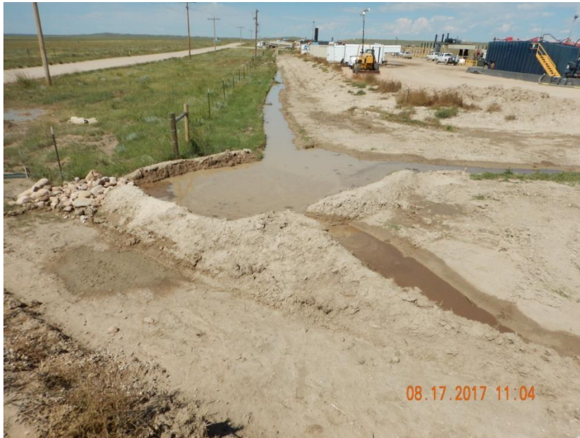
Photo 14. Photo taken from the southeast production facility pad, facing West. Appears the Operator has enlarged the sediment trap size. However, the sediment trap size could be enlarged because it appears flows have discharged over the embankment berms. Embankment material and embankment construction does not appear to be sufficiently compacted, as it appears unconsolidated material is contributing to sediment loss. Sediment trap outlet area does not appear to be properly constructed to capture outlet flows.
