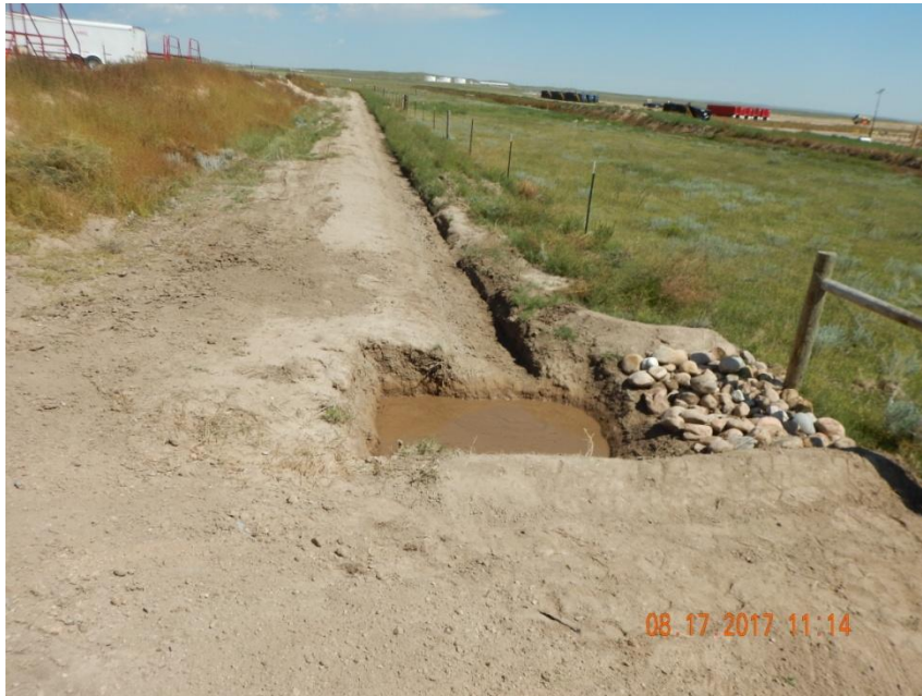
Photo 16. Photo taken from the west well pad, east entrance along the east side, facing North. Does not appear the sediment trap size has been enlarged. It appears the Operator has moved the position of the sediment trap outlet and constructed an embankment berm. However, embankment does not appear to be sufficiently compacted, as it appears unconsolidated material could be contributing to sediment loss.
