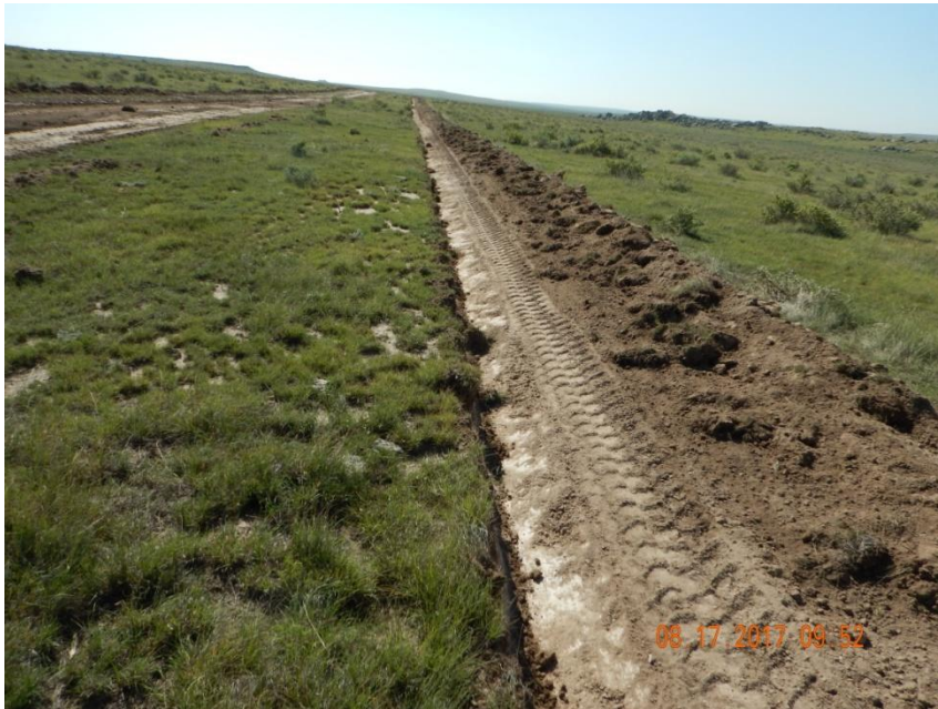
Photo 3. Photo taken from the southwestern location, facing Southeast. Topsoil salvage operations IN-PROCESS. Temporary BMP (i.e., ditch) installed around in the entire perimeter of the location.
