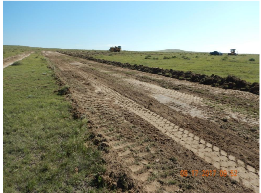
Photo 2. Photo taken from the northwestern location, facing Northeast. Topsoil salvage operations IN-PROCESS.
