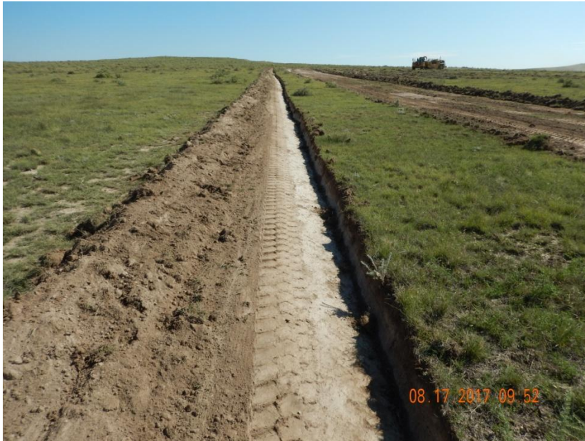
Photo 1. Photo taken from the northwestern location, facing Northeast. Topsoil salvage operations IN-PROCESS. Temporary BMP (i.e., ditch) installed around in the entire perimeter of the location.
