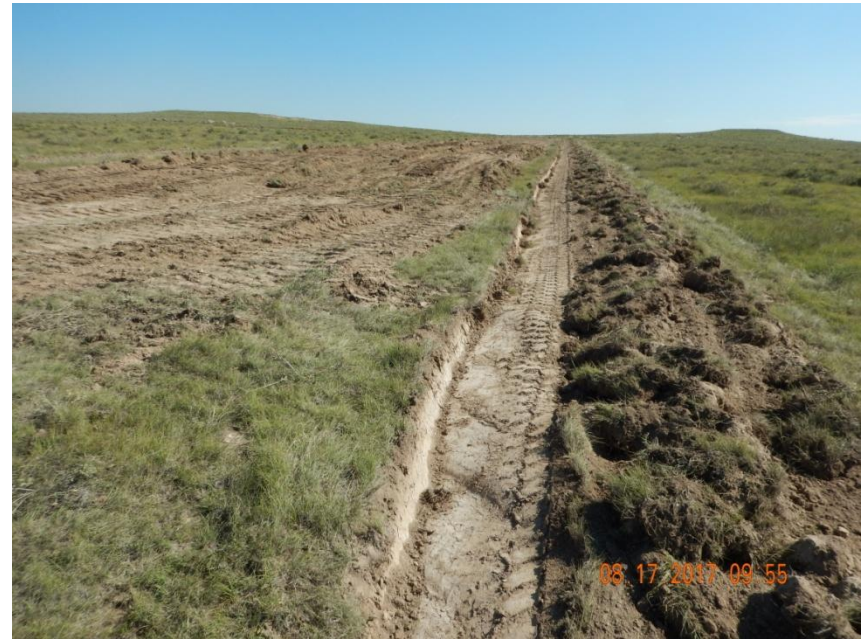
Photo 4. Photo taken from the southeastern location, facing Northeast. Topsoil salvage operations IN-PROCESS. Temporary BMP (i.e., ditch) installed around in the entire perimeter of the location. Topsoil stockpile being stored along the southeastern location.
