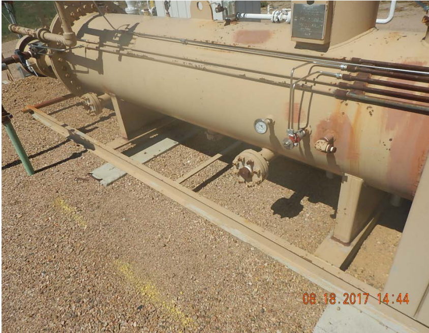
Photo 3: Separator not anchored
