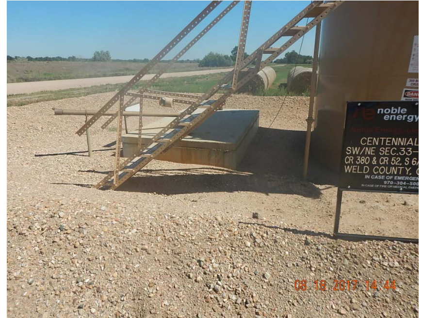
Photo 4: Concrete vault not anchored
