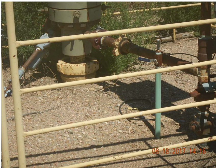
Photo 3: 1-1" riser at wellhead
