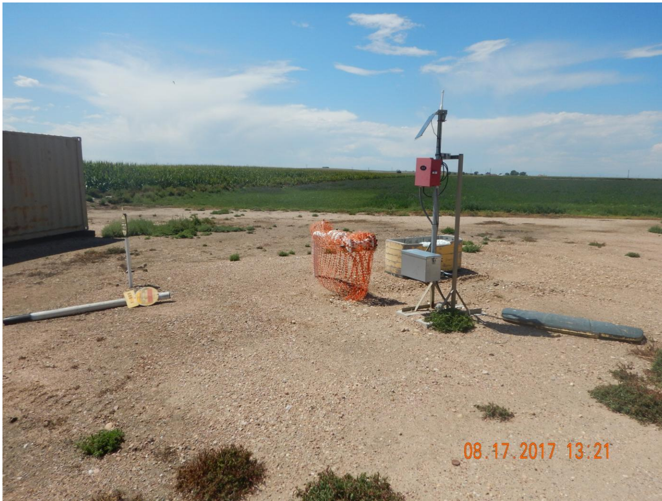
Photo 1: Photo taken from the battery location. Photo shows meter shed has been removed, however pipe equipment associated with the meter shed has not been removed. Photo also shows Battery location remains un-reclaimed
