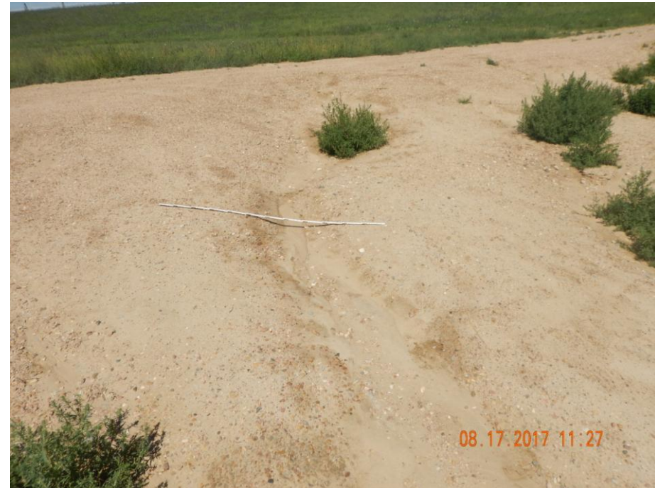
Photo 4: Photo shows gulley erosion continuing to form and degrade the location and access road. Inspection doc. #682502370 required operator to repair erosion and install/repair required BMPs. CA has not been addressed. 6 foot measuring stock for reference.
