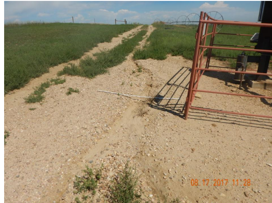
Photo 6: Photo shows gully erosion continuing to form and degrade the location and access road. Inspection doc. #682502370 required operator to repair erosion and install/repair required BMPs. CA has not been addressed. 6 foot measuring stock for reference.
