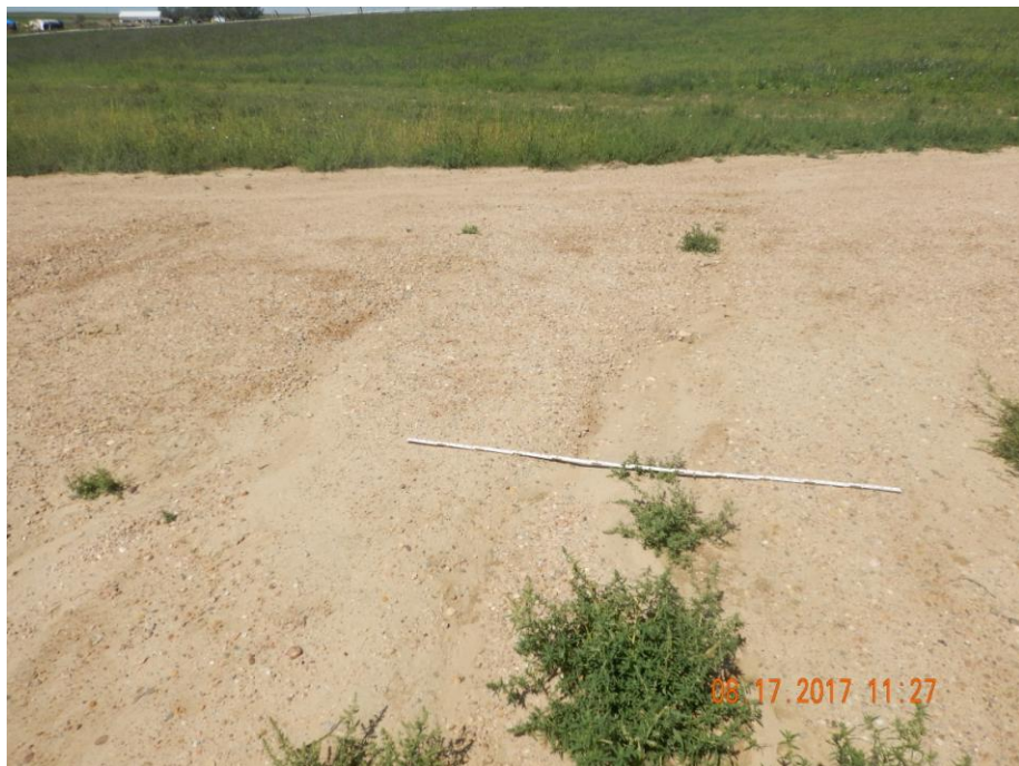
Photo 5: Photo shows gulley erosion continuing to form and degrade the location and access road. Inspection doc. #682502370 required operator to repair erosion and install/repair required BMPs. CA has not been addressed. 6 foot measuring stock for reference.
