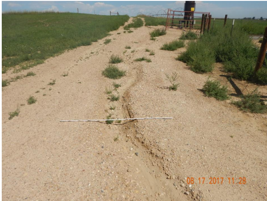
Photo 5: Photo shows gully erosion continuing to form and degrade the location and access road. Inspection doc. #682502370 required operator to repair erosion and install/repair required BMPs. CA has not been addressed. 6 foot measuring stock for reference.
