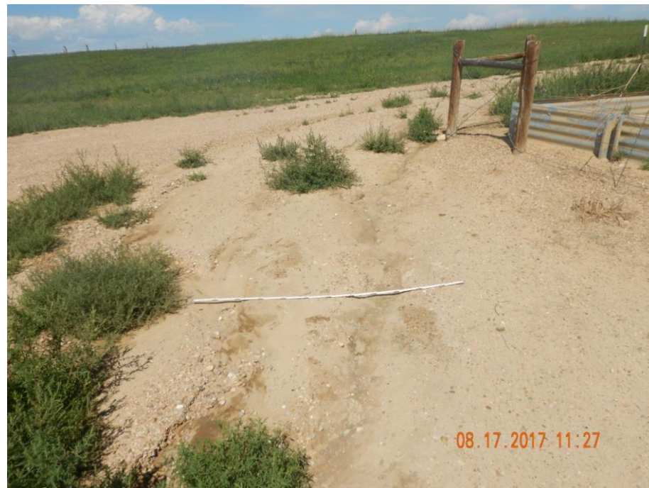
Photo 6: Photo shows gulley erosion continuing to form and degrade the location and access road. Inspection doc. #682502370 required operator to repair erosion and install/repair required BMPs. CA has not been addressed. 6 foot measuring stock for reference.
