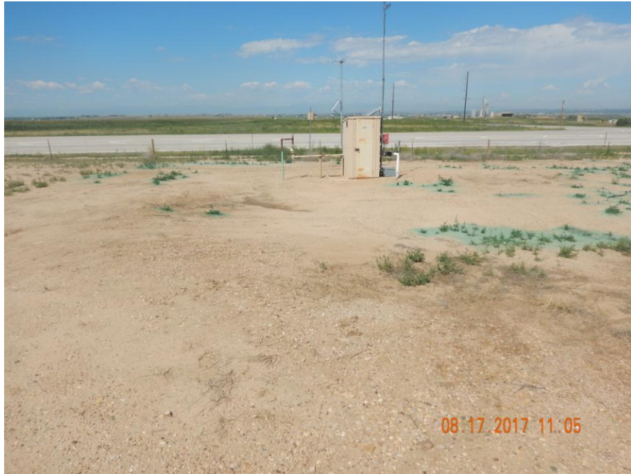
Photo 2: Photo taken from the former battery location. Photo shows meter shed remains, and location remains un-reclaimed.
