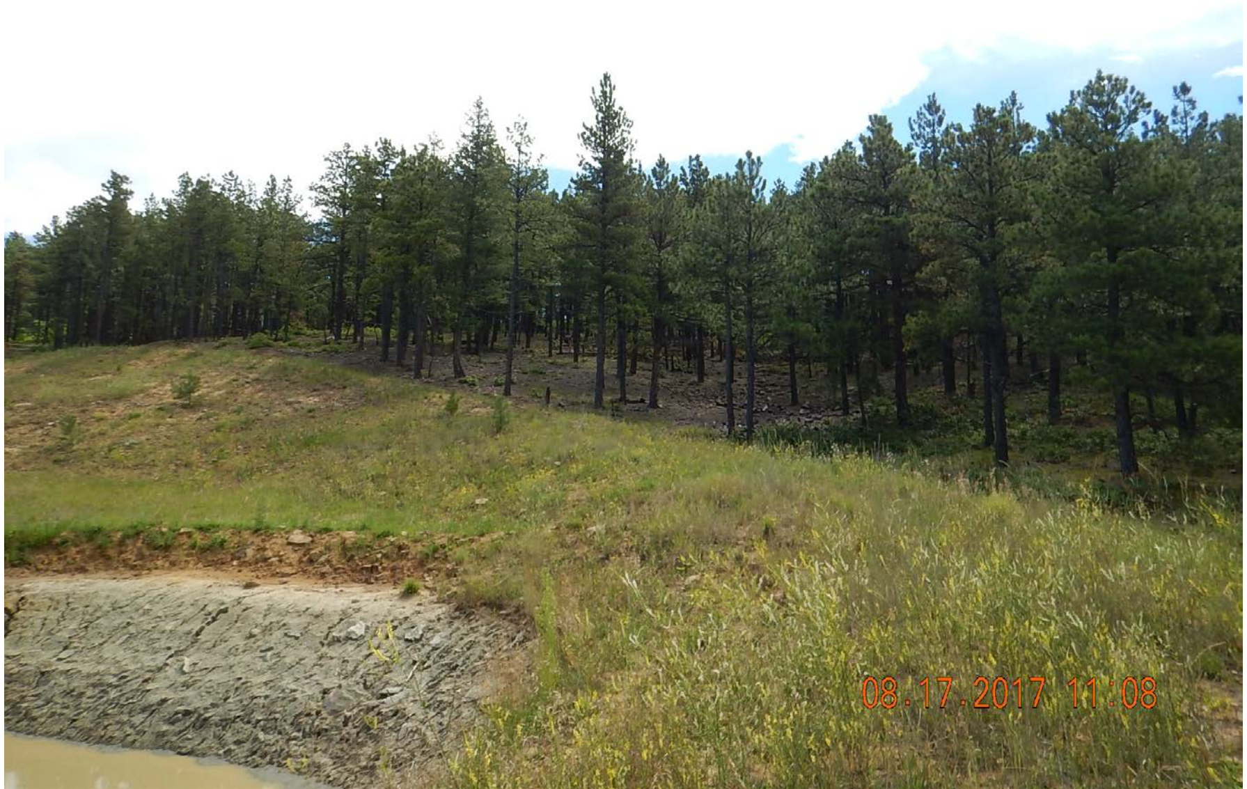
Example of the condition of trees on the east side of the pit.
