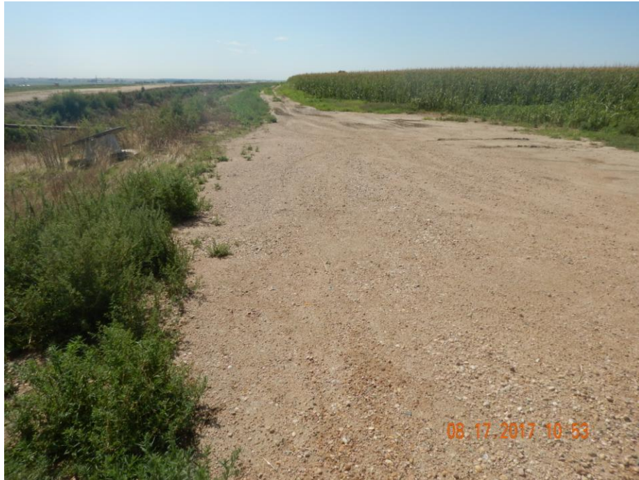
Photo 2: Photo taken from the east end of the battery location, facing south. Photo shows battery location and access road remains un-reclaimed.
