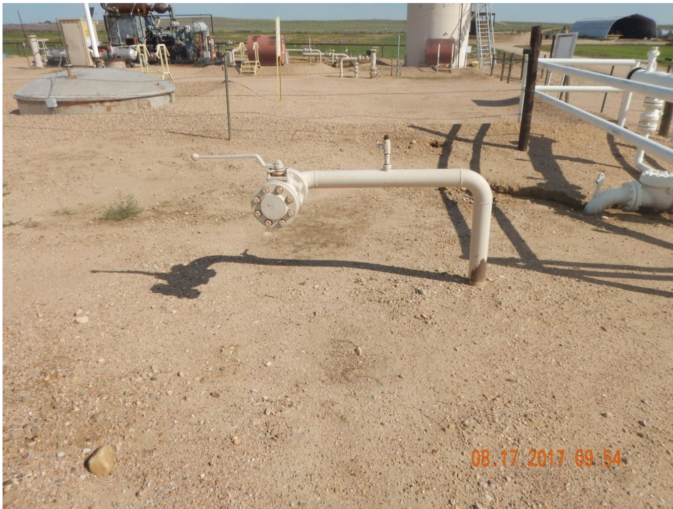
Photo 2: Photo taken from the battery facility, facing north. Photo shows riser that was once related to the meter sheds remain.
