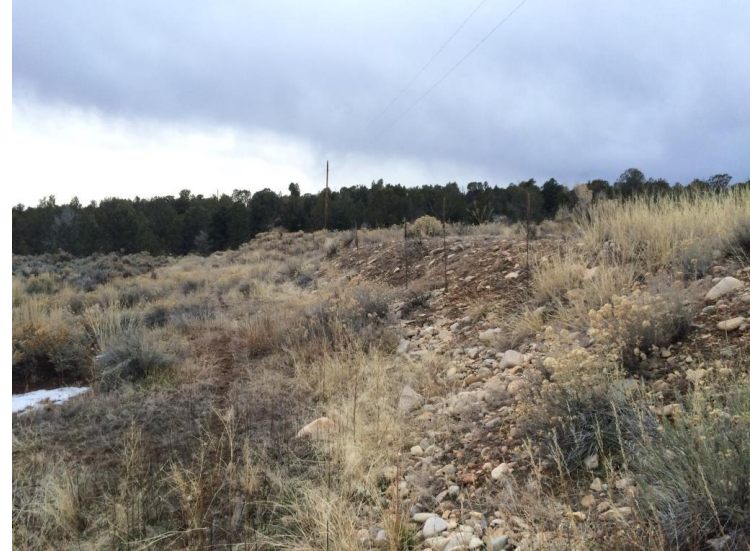
Photo 6 – Looking south along fill slope.
