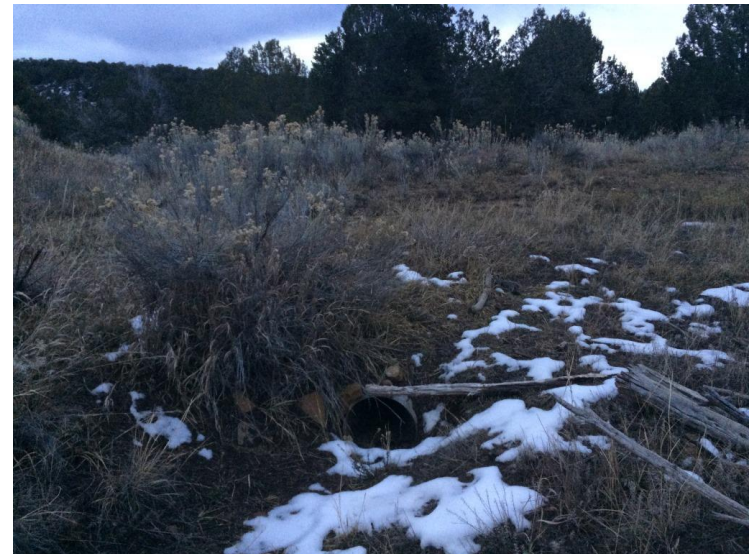
Photo 8 – Looking east toward culvert in access road.
