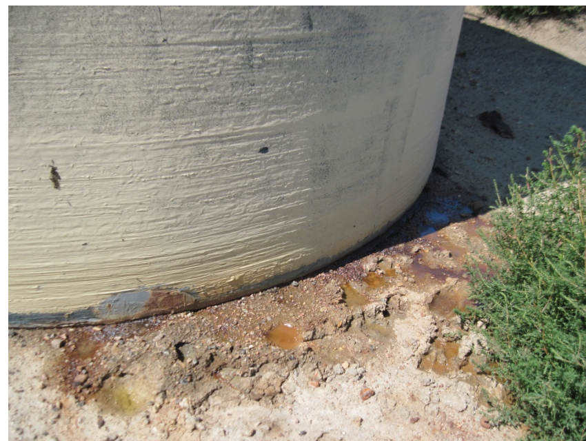
WATER TANK LEAK AND WEEDS
