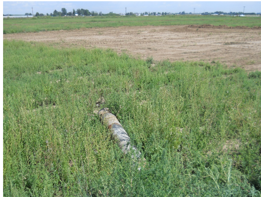
Cut surface casing west edge of PA location
