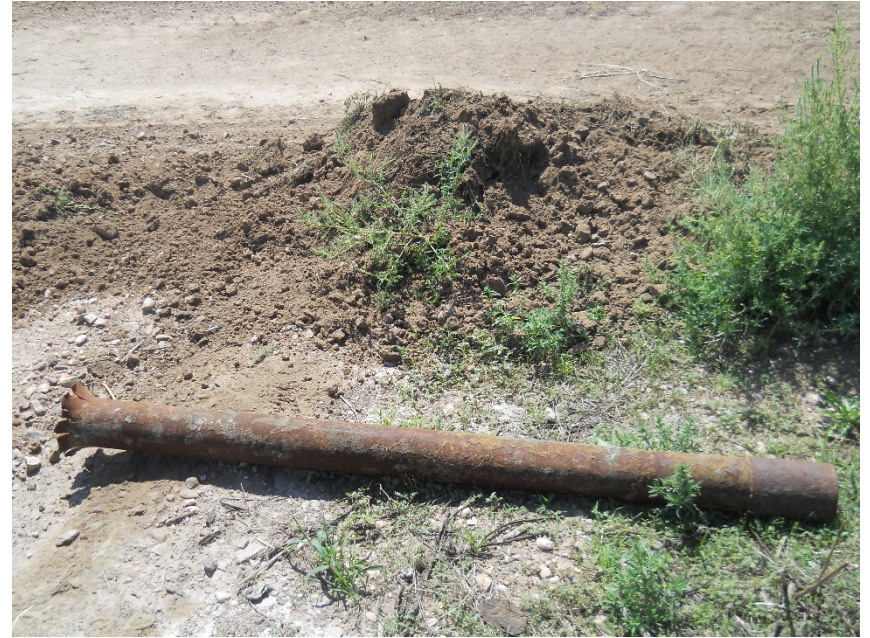
Cut casing west edge of PA location
