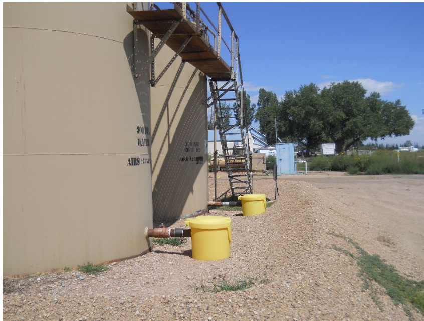
Tank battery looking north
