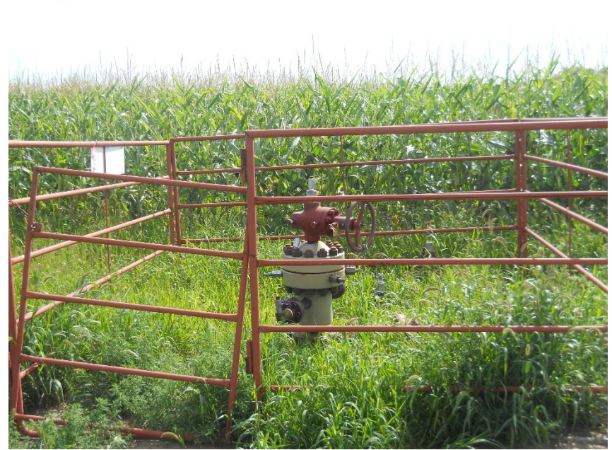
Wellhead looking east, Christiansen 35-15
