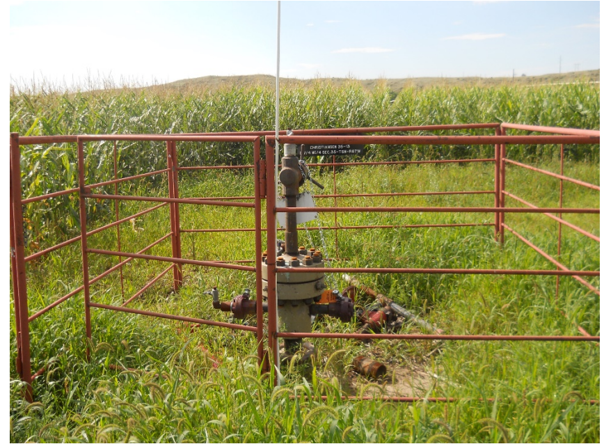
Wellhead looking south, Christiansen 35-13. Actively growing weeds need to be controlled
