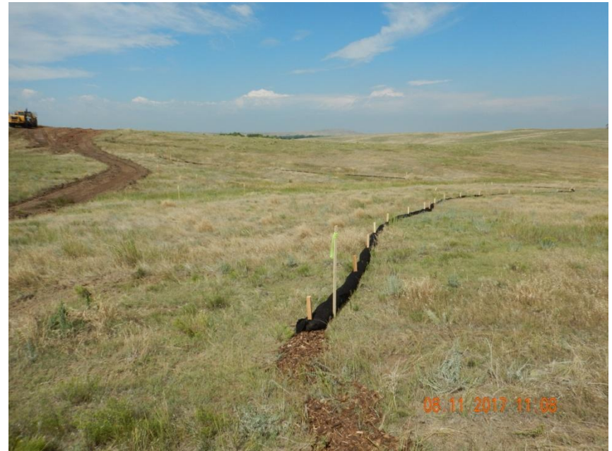
Photo 4. Photo taken from the southwestern location, facing West. Topsoil salvage operations IN-PROCESS. Temporary BMP (i.e., filtrex wattle) installed around in the perimeter of the location.
