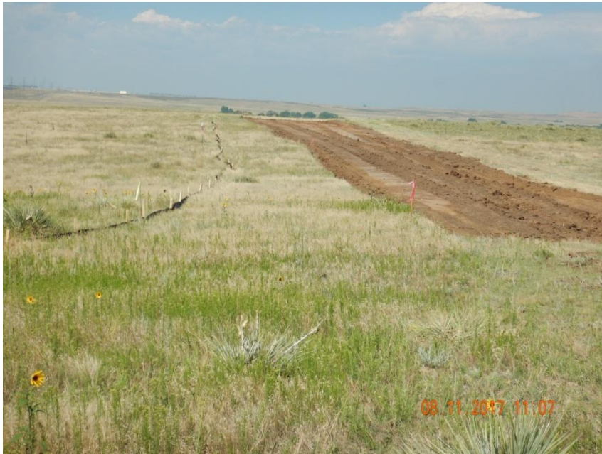
Photo 3. Photo taken from the southeastern location, facing West. Topsoil salvage operations IN-PROCESS. Temporary BMP (i.e., filtrex wattle) installed around in the perimeter of the location.
