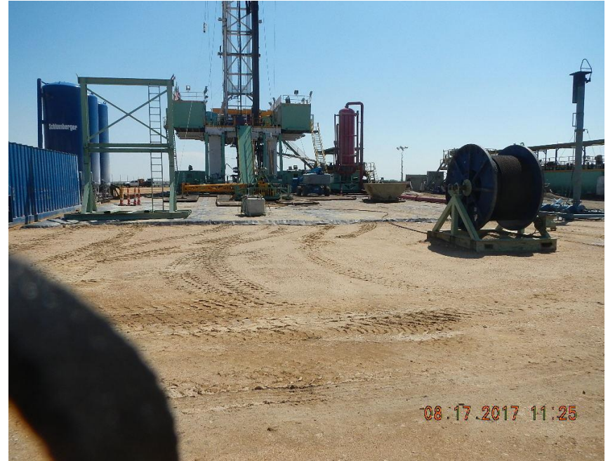
Photo 4: Mats and lining under drilling operations.
