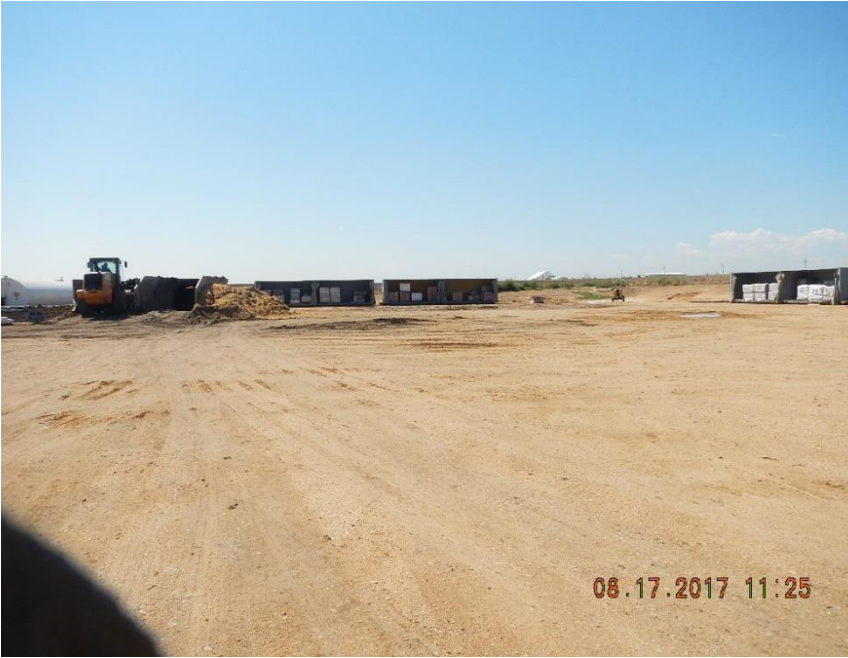
Photo 5: Materials stored under conex
