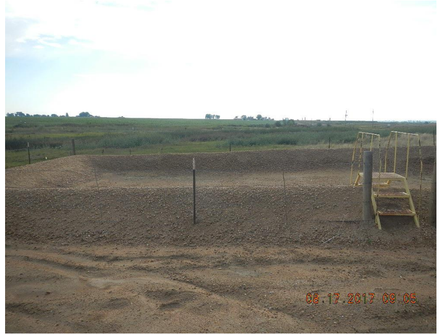
Photo 6: Weed debris has been removed from within berm.
