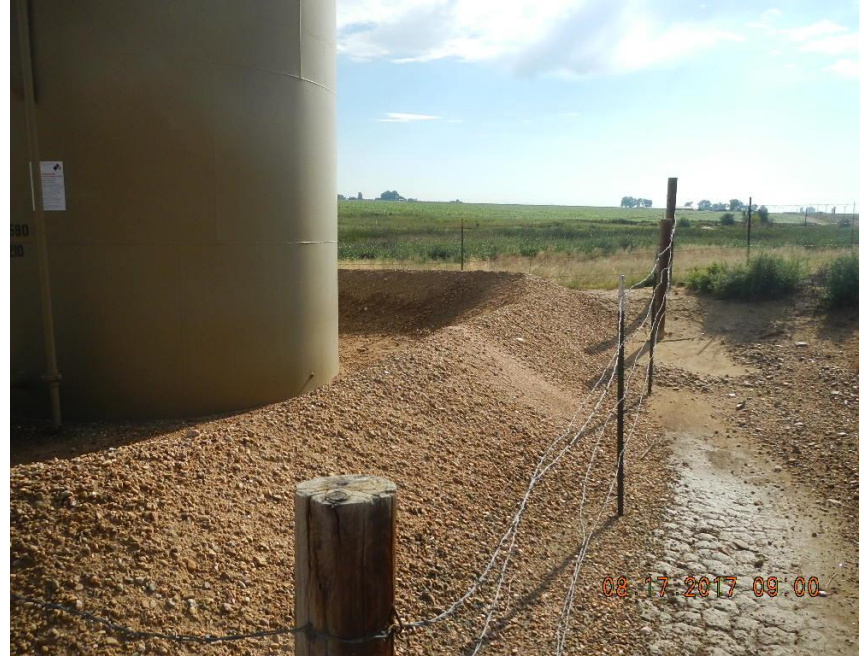
Photo 4: Berm has been repaired.
