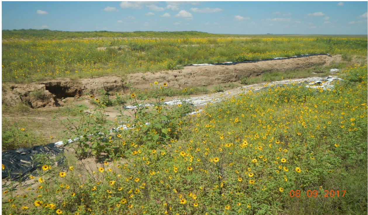
photo 3: There is a pit at the east side of the location which has torn liner debris.
