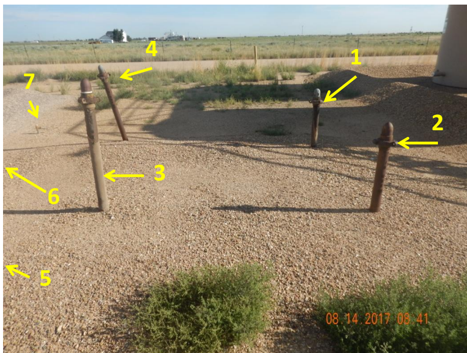
Photo 3: Photo taken from the central area of the battery facility, facing north. Photo shows risers at the battery. Inspection doc. #682502037 required operator to comply with reclamation requirements and the 2017 Flowline NTO to remove the risers. Operator appears to have only sprayed "In Use" on five (5) of the seven (7) risers visible (risers labeled 1-5). Risers labeled "In Use" will require pressure testing.
