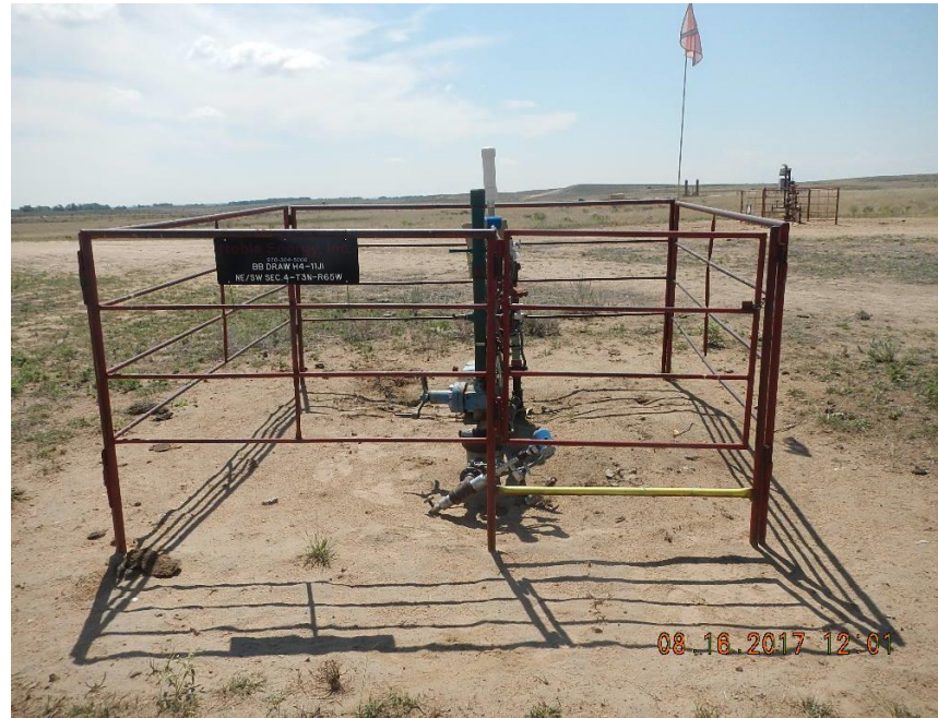
Photo 2: Current inspection. Contact company with phone number and weeds addressed.
