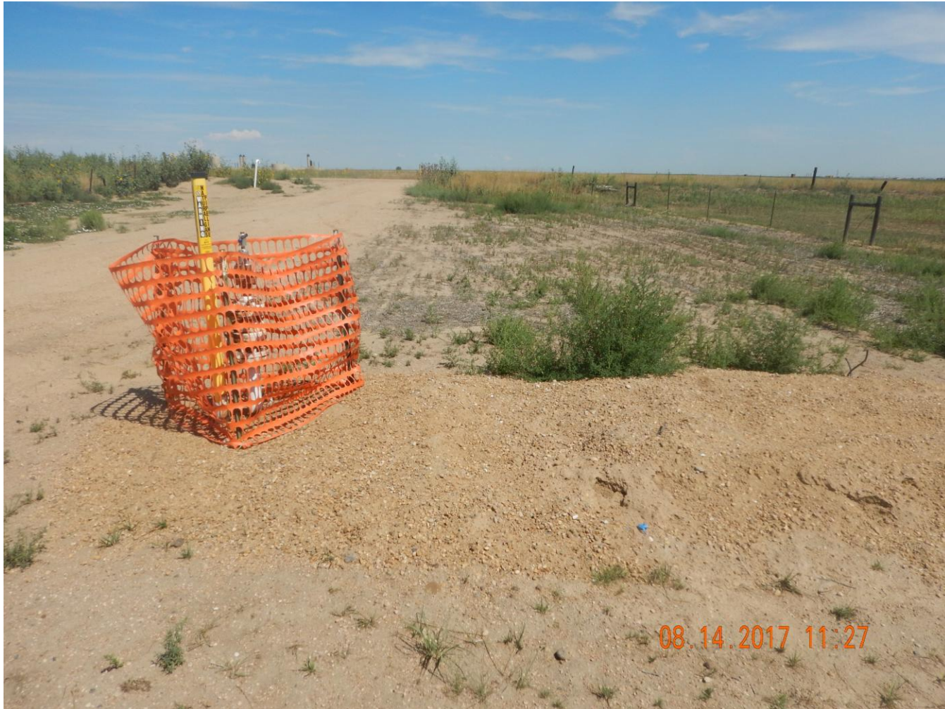
Photo 1: Photo taken from the south end of the battery location. Photo shows meter shed has been removed, however pipe riser has not been removed. Riser is now subject to reclamation requirements for removal.
