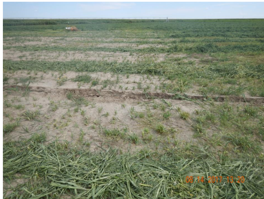
Photo 8: Photo taken from the south end of the battery location, facing east. Noble indicated surface owner seeded a “sudax grass” into the disturbance area after the previous inspection. Photo shows vegetation appears to have had difficulty establishing on large portions of the disturbance area, as establishment was not uniform and large areas of the location do not show sign that any germination had occurred, and remain predominantly bare and unvegetated.
