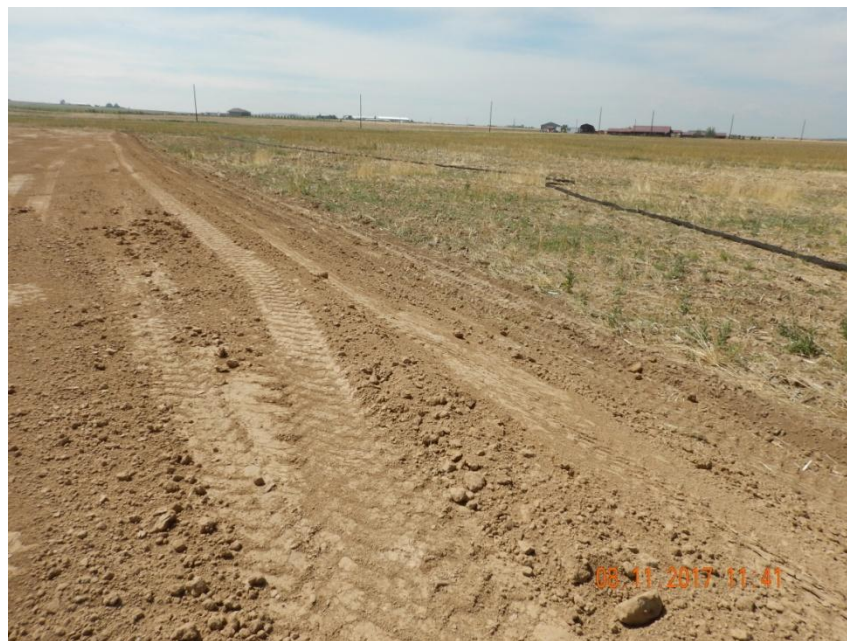
Photo 2. Photo taken from the western location, facing South. A temporary BMP (filtrexx wattle) has been installed around the entire perimeter of the location. Appears there is a vegetative buffer between the western disturbance area and the BMP to aid in stormwater controls.
