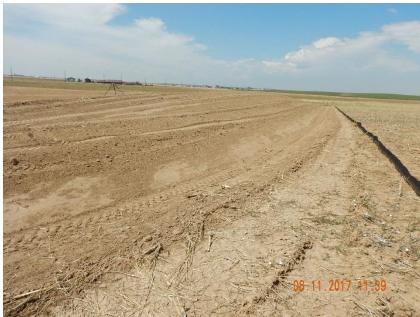
Photo 1. Photo taken north of the topsoil stockpile, facing West. A temporary BMP (filtrexx wattle) has been installed around the entire perimeter of the location.
