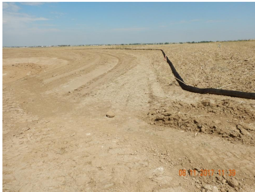
Photo 4. Photo taken from the entrance of location, facing North. A temporary BMP (filtrex wattle) has been installed around the entire perimeter of the location.
