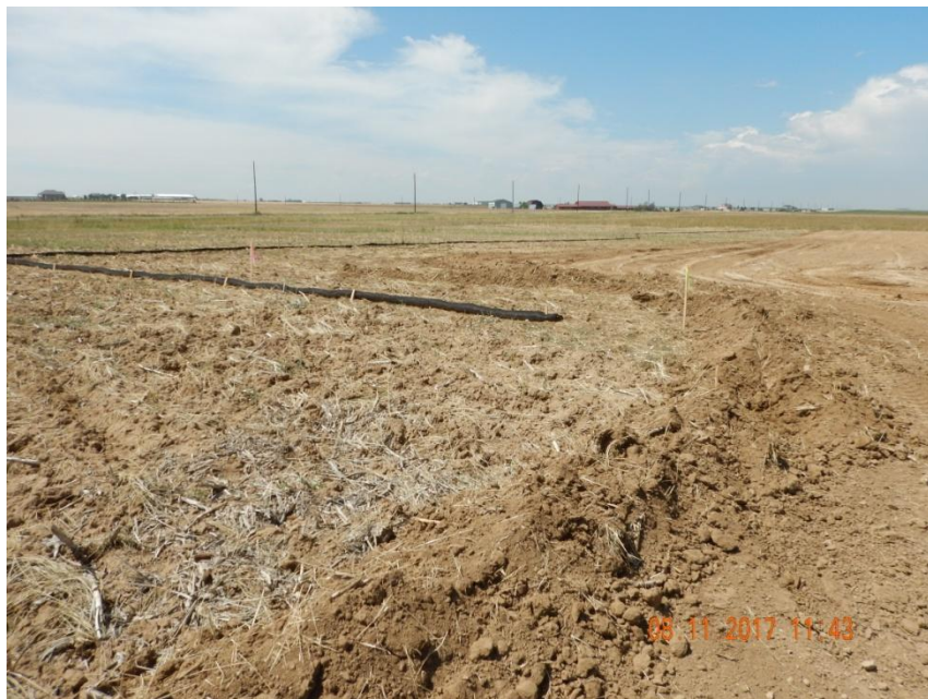
Photo 3. Photo taken from the entrance of location, facing Southwest. A temporary BMP (filtrex wattle) has been installed around the entire perimeter of the location. Appears there is a vegetative buffer between the southern disturbance area and the BMP to aid in stormwater controls.
