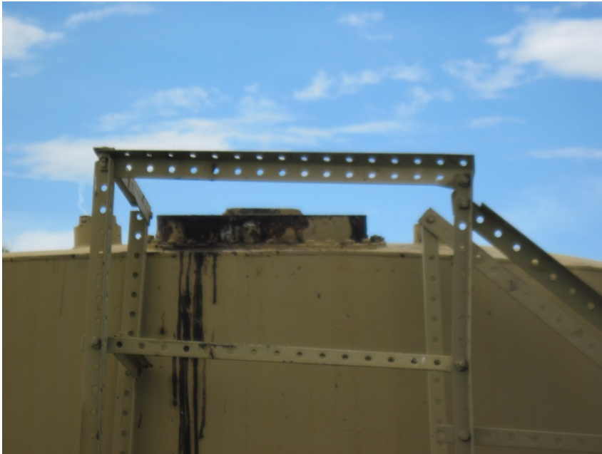
NO THIEF HATCH ON PROD TANK
