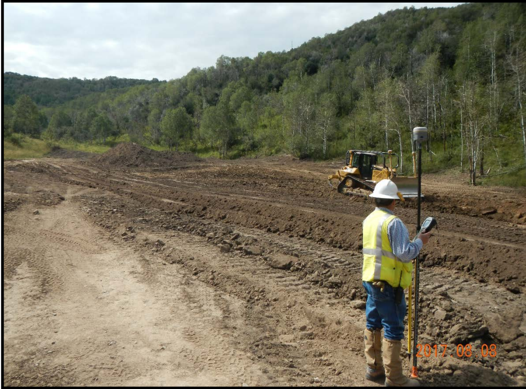
Terrace #1. Adding top soil and contouring.
