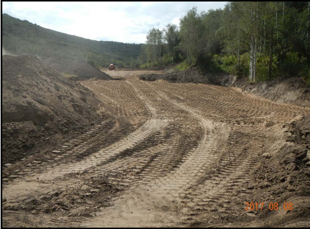
Looking uphill from Terrace #6 toward Terrace #3. Terraces excavated, sampled and backfilled.
