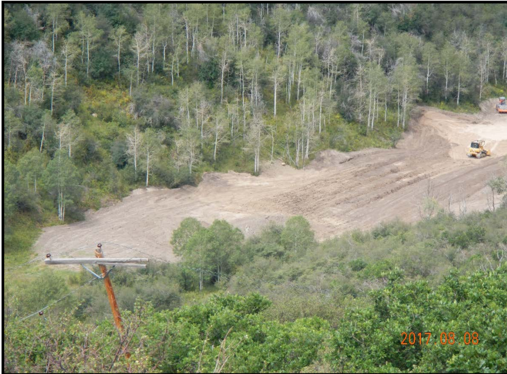
View of the Terrace #1, excavated, sampled and back filled. Currently leveling and adding top soil.
