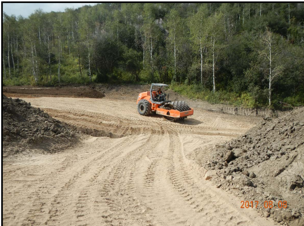
Compacting soil in terraces
