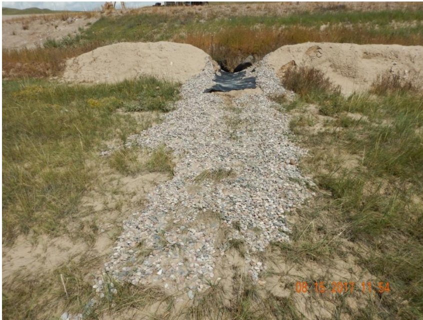
Photo 7. Photo taken from the southeast sediment trap outlet area, facing North. Sediment trap does not appear to have a sufficient stabilized outlet. Rock material does not appear to be the appropriate size and the plastic-like material only appears to allow stormwater flows to accelerate out of the sediment trap.
