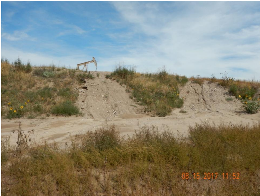
Photo 5. Photo taken west of the entrance to the location, facing North. Gully erosion is forming and rill erosion observed along the fill slope.
