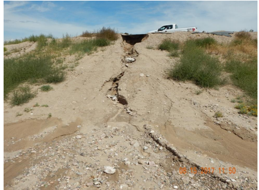
Photo 2. Photo taken from the southwestern location, facing North. Gully erosion observed along the fill slope. Photo illustrates sediment deposition accumulation.
