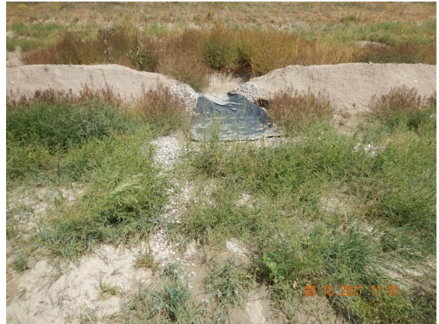
Photo 4. Photo taken from the southwest sediment trap outlet area, facing North. Sediment trap does not appear to have a sufficient stabilized outlet. Rock material does not appear to be the appropriate size and the plastic-like material only appears to allow stormwater flows to accelerate out of the sediment trap. A point of sediment discharge was observed south of the outlet area.
