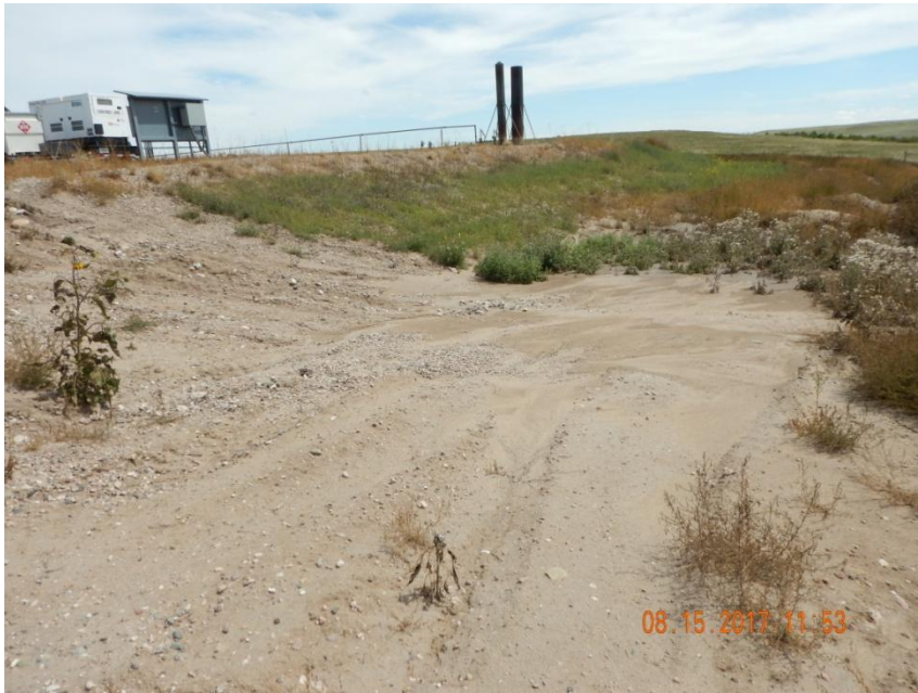
Photo 5. Photo taken east of the entrance to the location, facing East. Photo illustrates sediment deposition accumulation and in need of maintenance.
