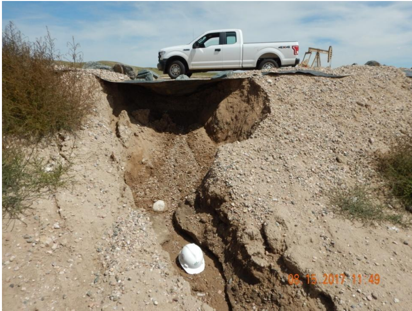
Photo 1. Photo taken from the southwestern location, facing North. Gully erosion observed along the fill slope.
