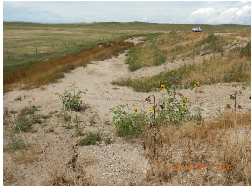
Photo 6. Photo taken from west of the entrance to the location, facing West. Photo illustrates sediment deposition accumulation and in need of maintenance.
