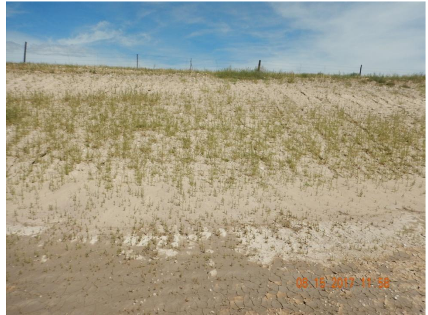
Photo 8. Photo taken from the northern cut slope, facing North. Rill erosion observed throughout the cut slope, except for the northeast corner where sediment blankets were installed.
