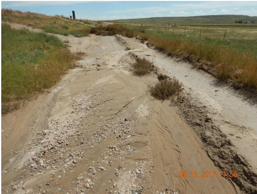
Photo 3. Photo taken from the southwestern stormwater management area, facing East. Photo illustrates sediment deposition accumulation and in need of maintenance.
