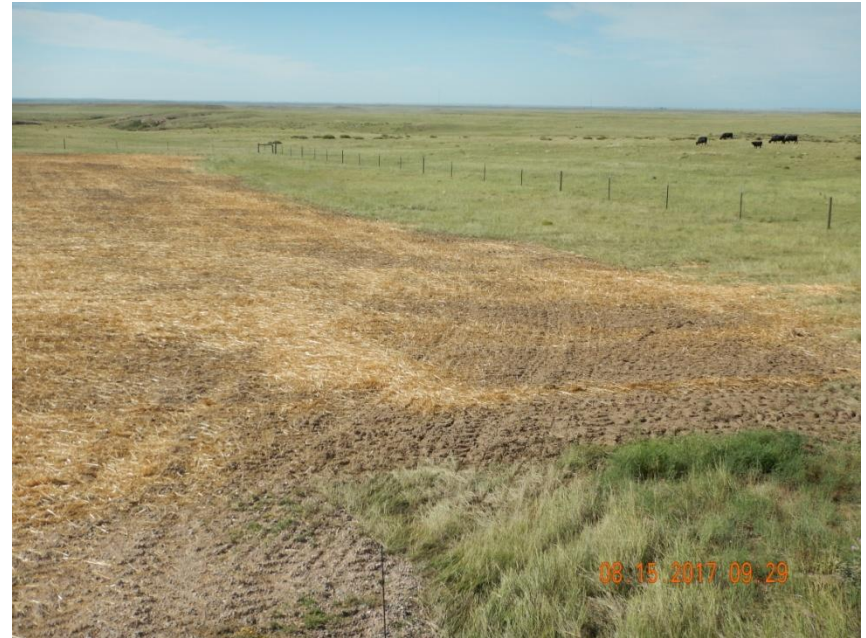
Photo 4. Photo taken from the entrance of location, facing Southwest. Interim reclamation activities have been performed and are in process. Appears erosion controls have been installed to stabilize the seeded soil. Did not observe any germination throughout the interim area.
