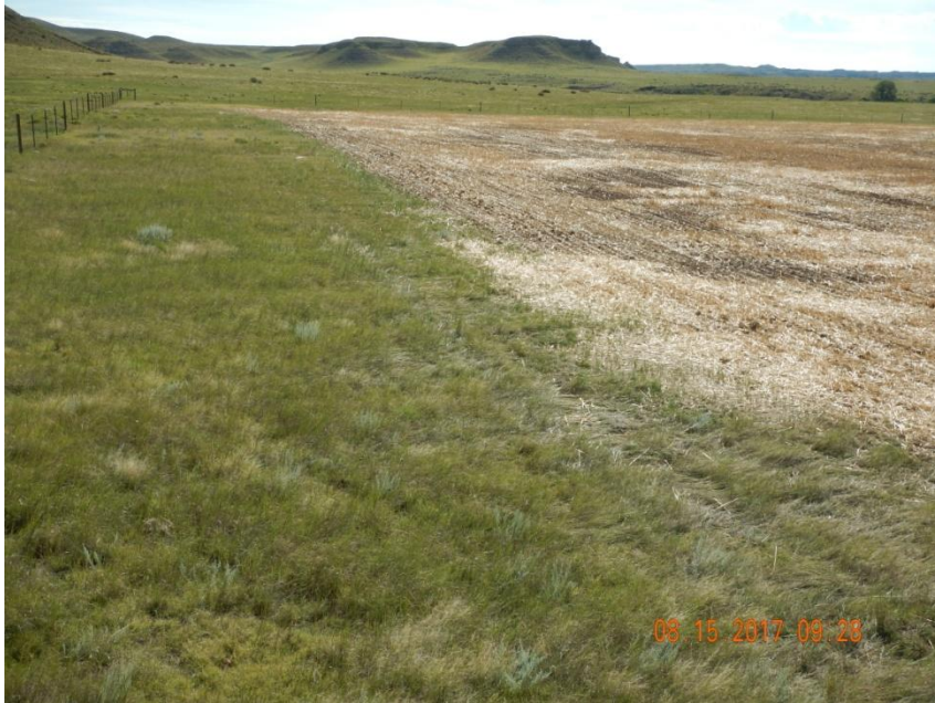
Photo 1. Photo taken from the entrance of location, facing East. Interim reclamation activities have been performed and are in process. Appears erosion controls have been installed to stabilize the seeded soil. Did not observe any germination throughout the interim area.
