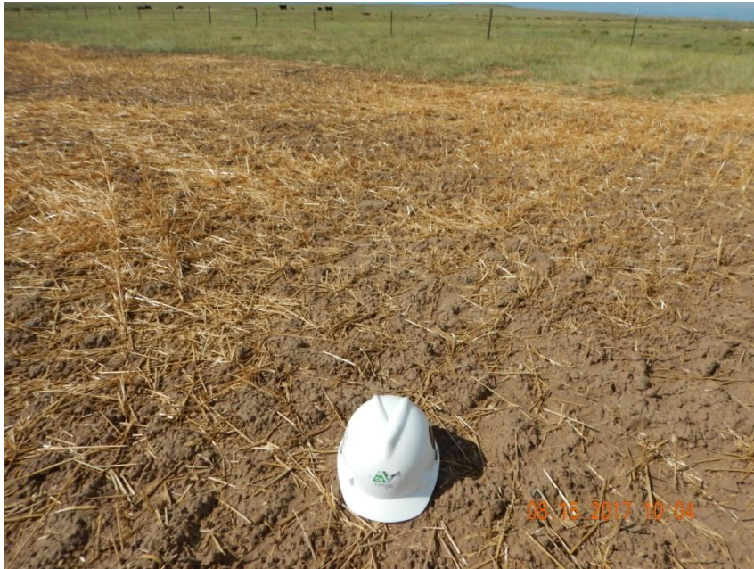
Photo 5. Photo taken from the western interim area, facing West. Appears erosion controls have been installed to stabilize the seeded soil. Did not observe any germination throughout the interim area.
