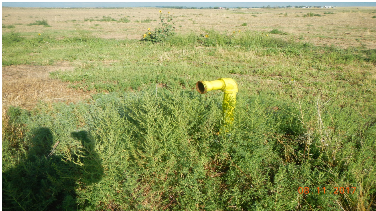
photo 1: A section of the pipe riser has been removed since the previous inspection. The remaining riser has been painted fluorescent. Lat/Long:39.98959,-104.54693
