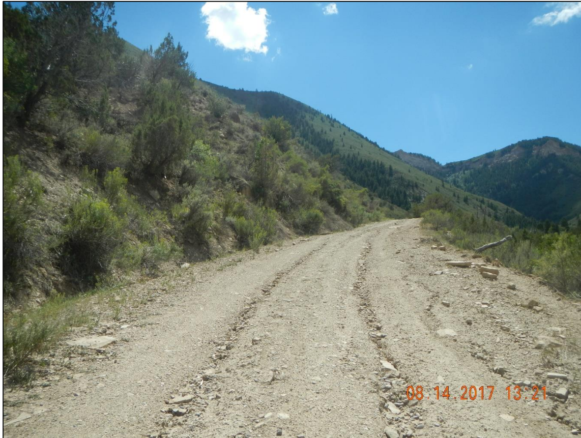
Erosion of access road and sediment build up in ditch.
