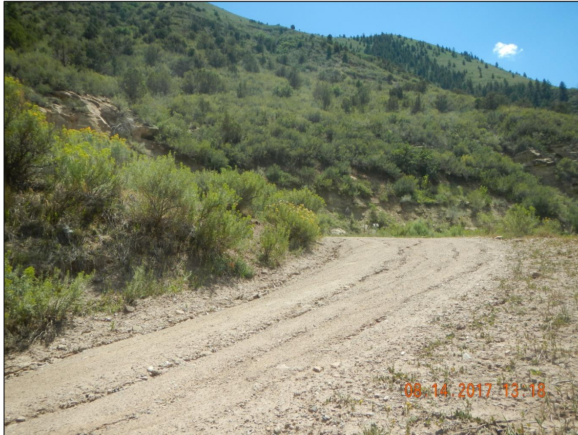
Erosion of access road at entrance of location
