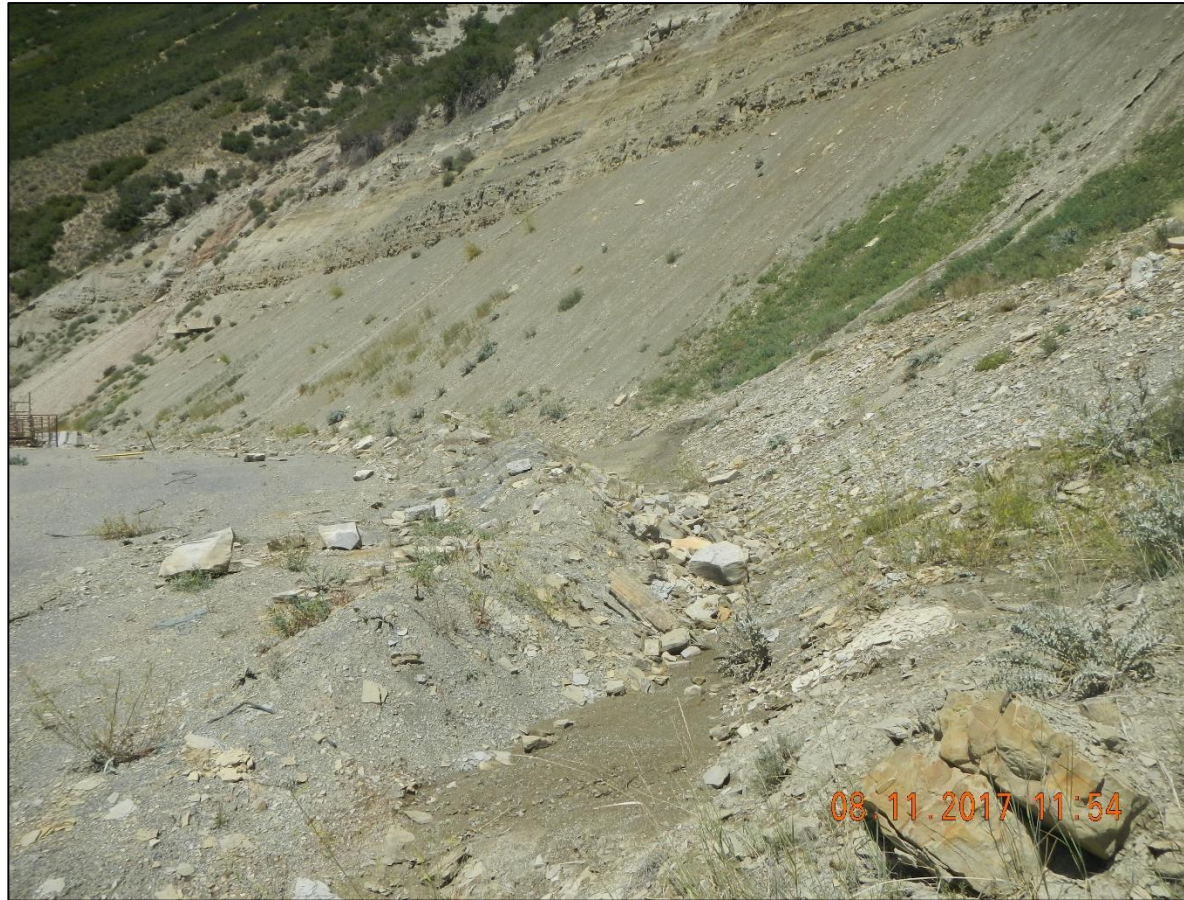
Sediment build up in ditch along cut slope wall.
